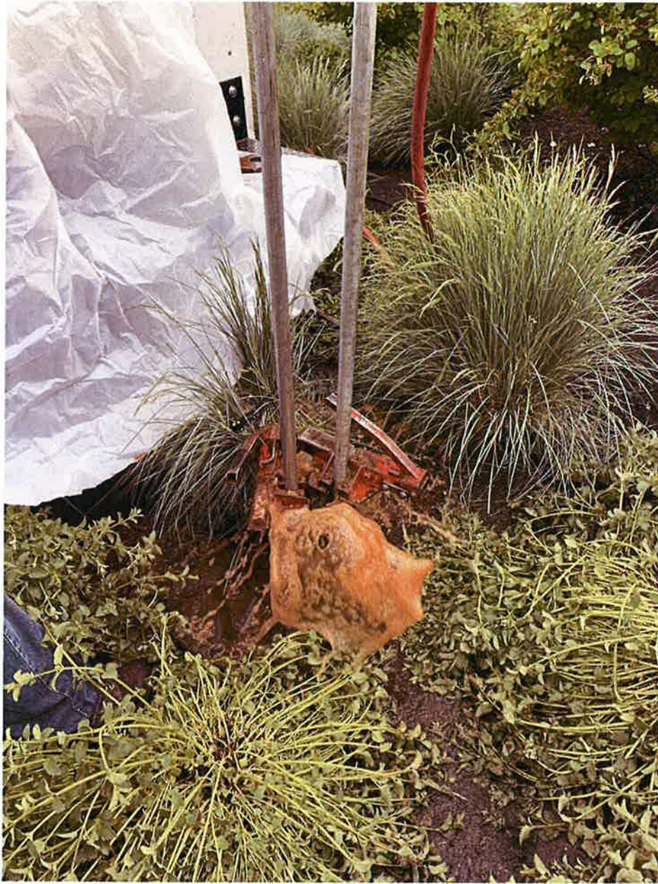
Figure 1: Production Well Being Cleared of Sands and Clays.
