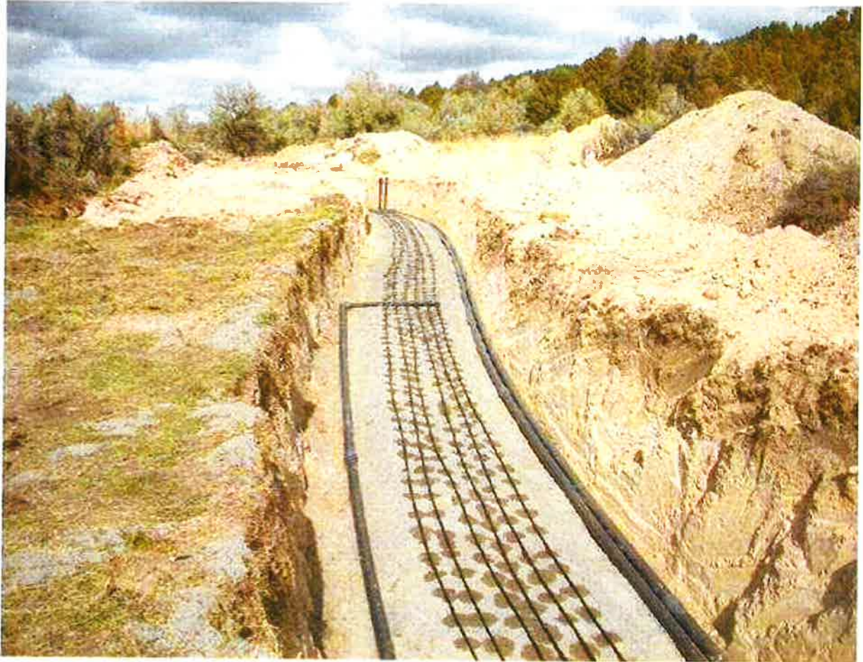
Lower Ground Bed Cathodic Protection Drip Line in Open Trench during Construction
