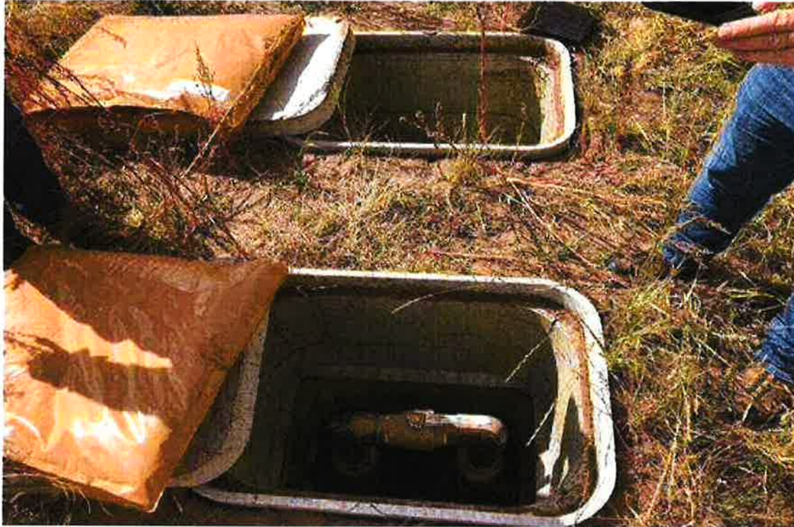
Upper Ground Bed Blowoff Box at Northeast Corner of Ground Bed
