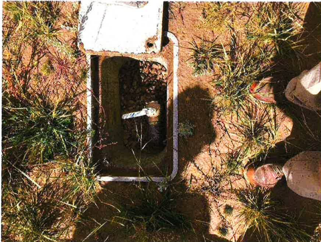
Upper Ground Bed Blowoff Box at Northeast Corner of Ground Bed
