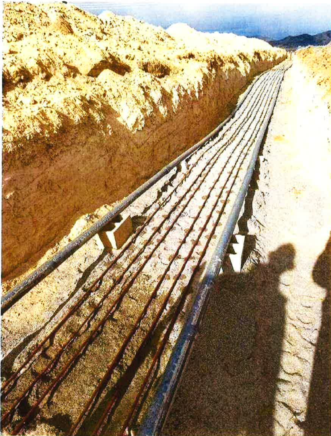
Upper Ground Bed Cathodic Protection Drip Line in Open Trench during Construction
