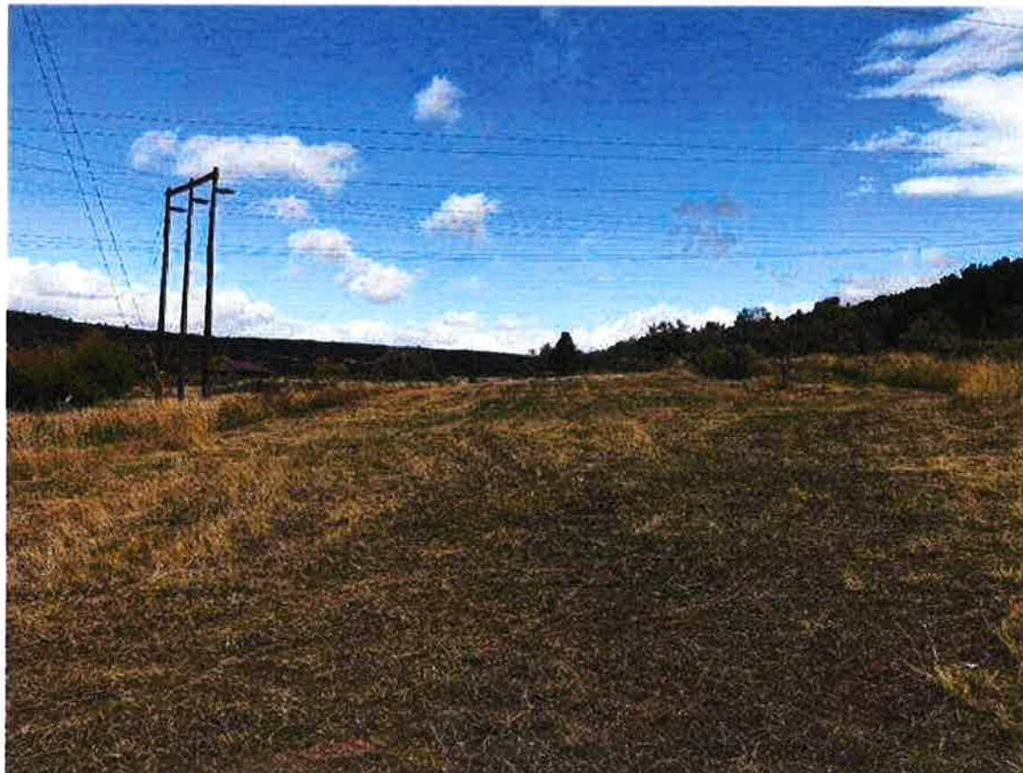
Lower Cathodic Protection Ground Bed, Viewing North
