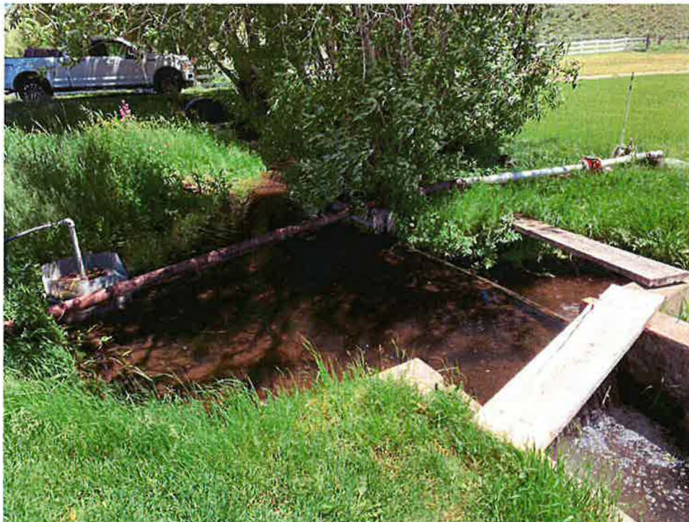
Figure 8: Southern Red Pump Meter on South (right side) side of Seamans Creek.
