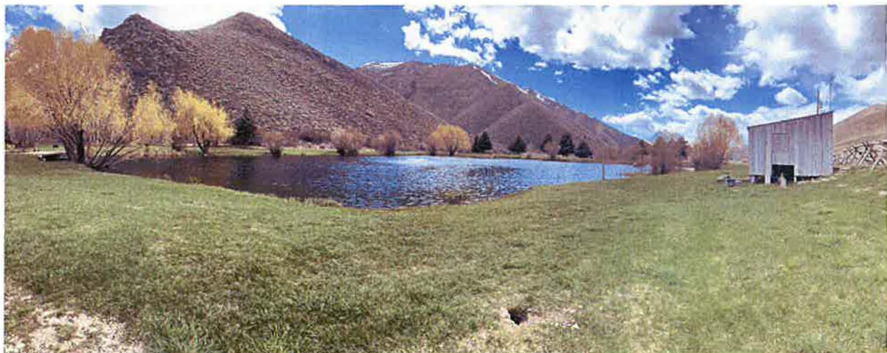
Figure 2: Pump Pond Panorama Looking Southwest from North Bank.
