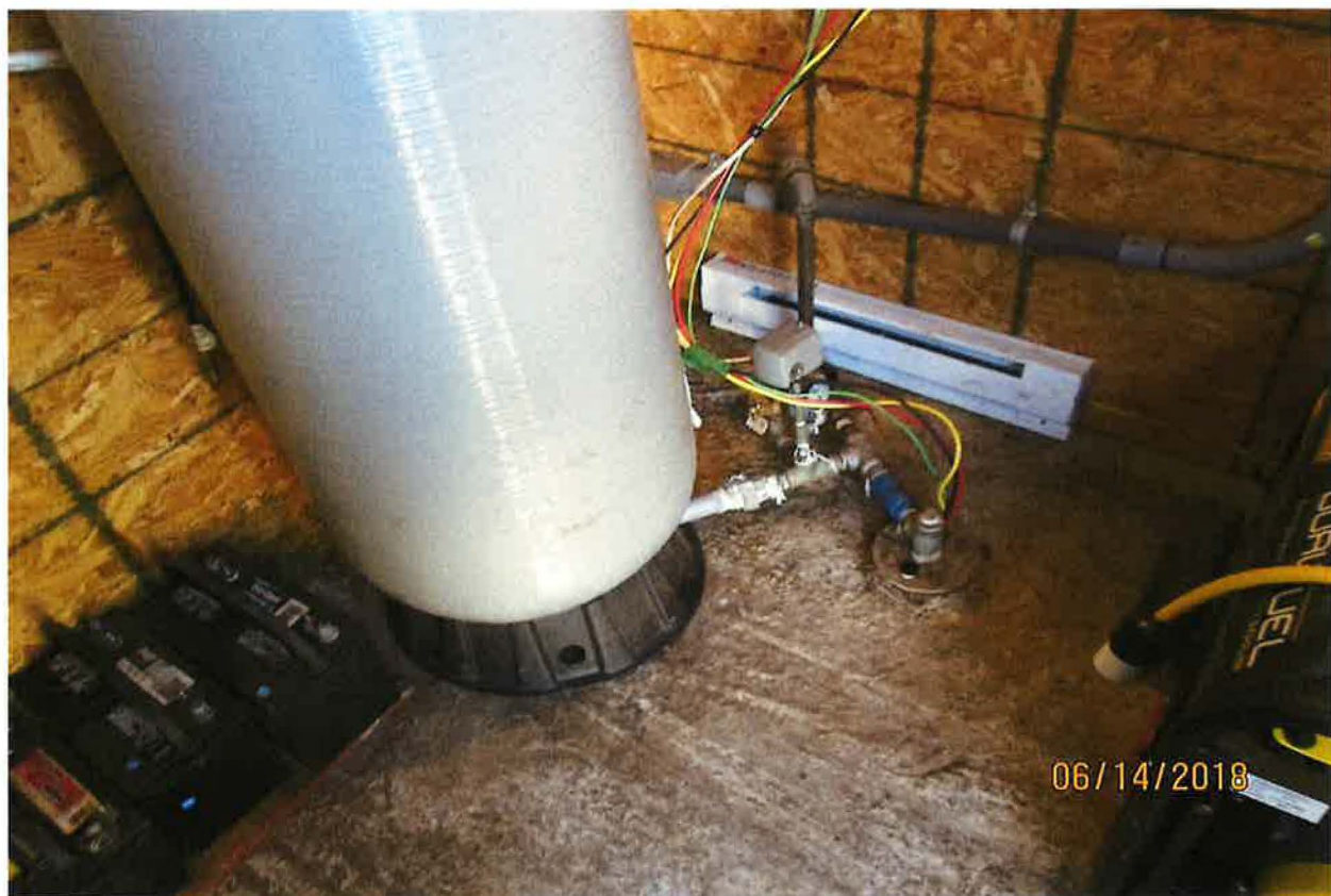
Well located next to pressure tank. No proper location to conduct measurement. Theoretical pumping equation and pump curve estimate around 8 gpm.
