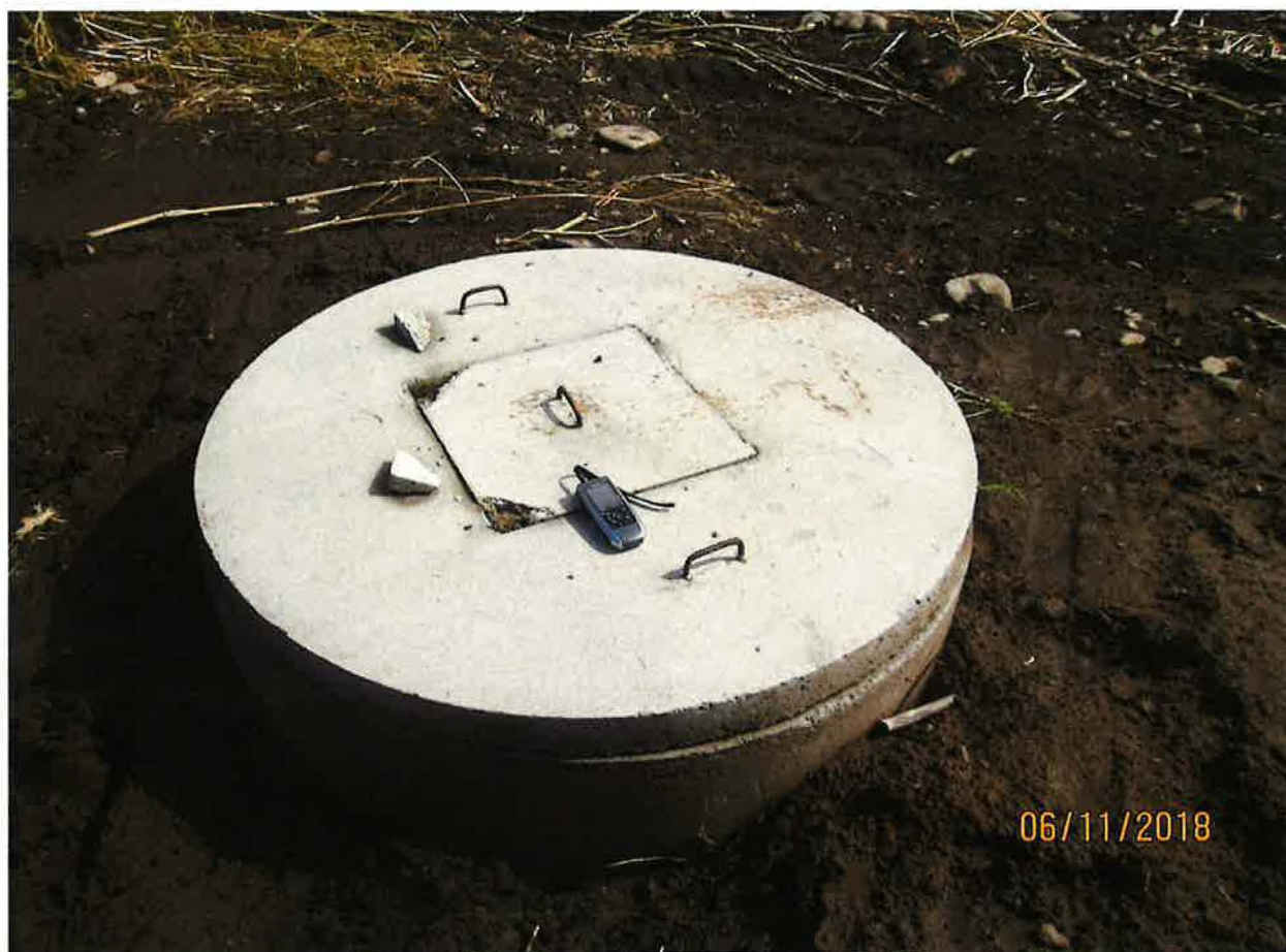
Spring POD with concrete cistern.
