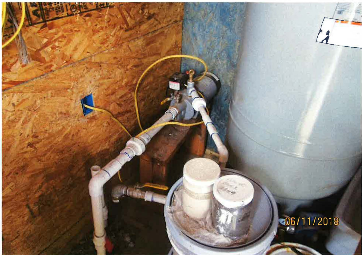
Inside pump house with pressure tank and pump. House was located a good distance away and required pump because of the distance.
