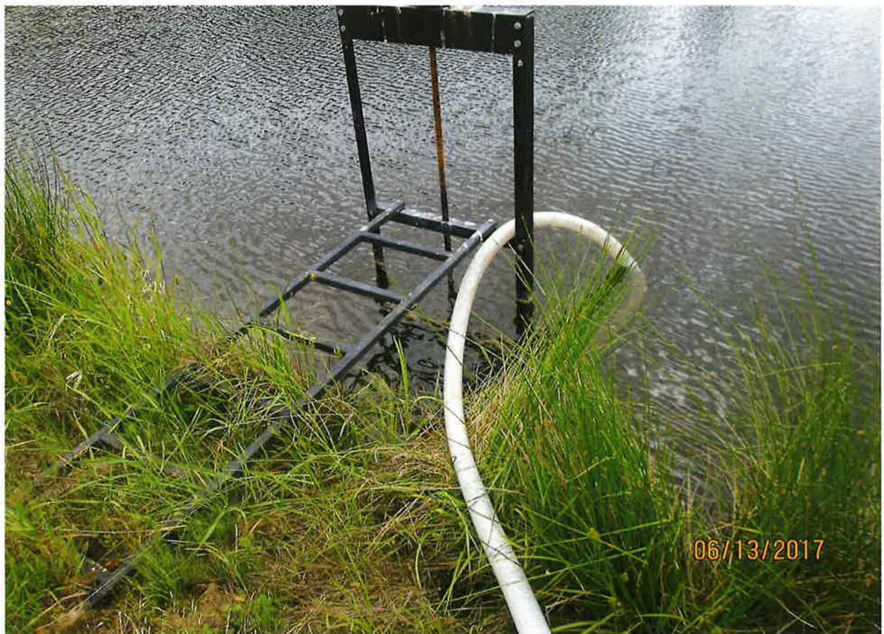
POD FROM POND & POND HEADGATE
