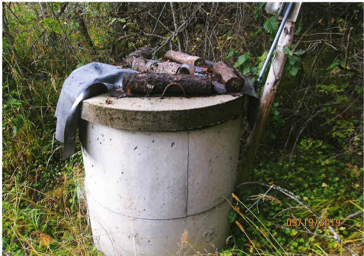
POD – HAND DUG WELL
