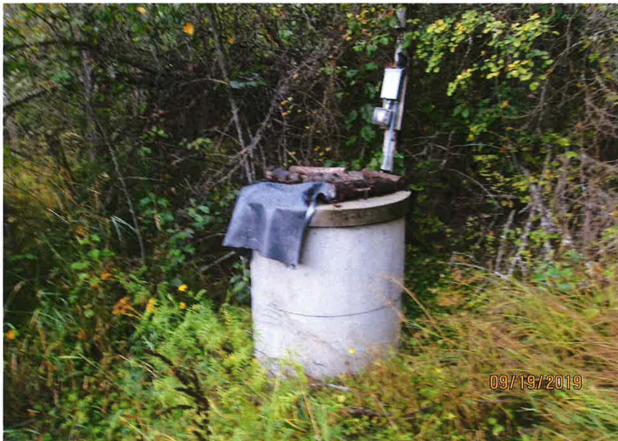
POD – HAND DUG WELL
