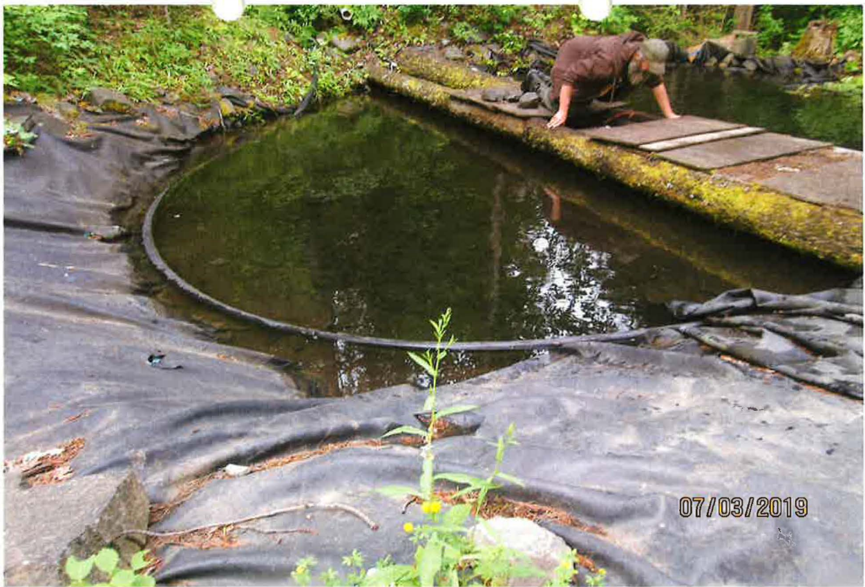
24HR CATCH BASIN AT POD
