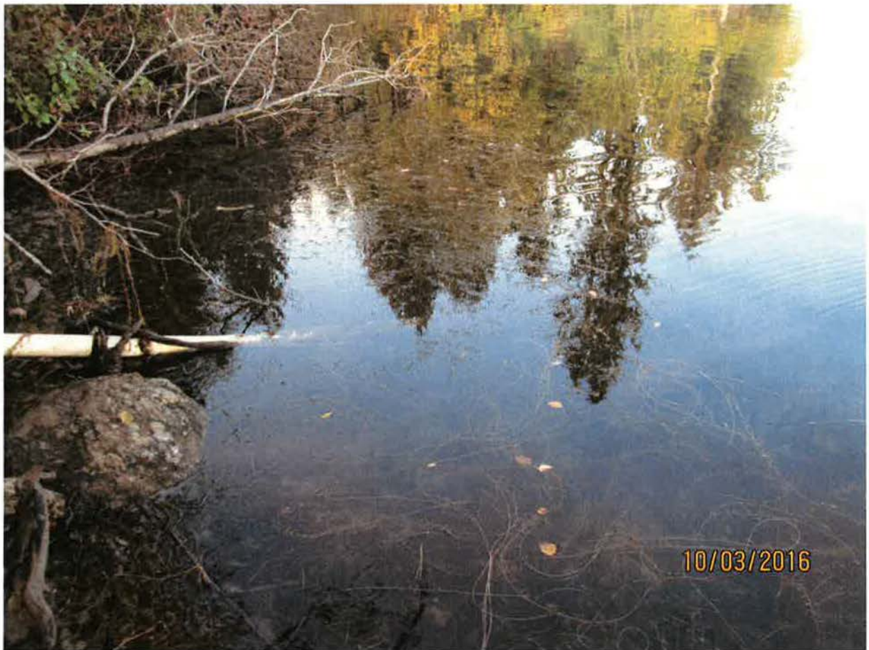
Intake pipe going into river.
