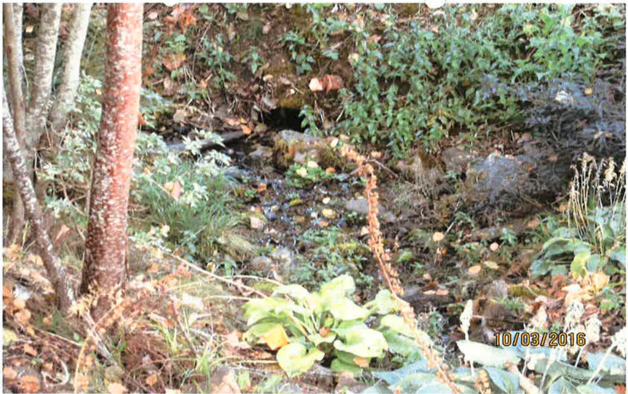
Waterline to pond going through culvert of unnamed stream where pond flows out.
