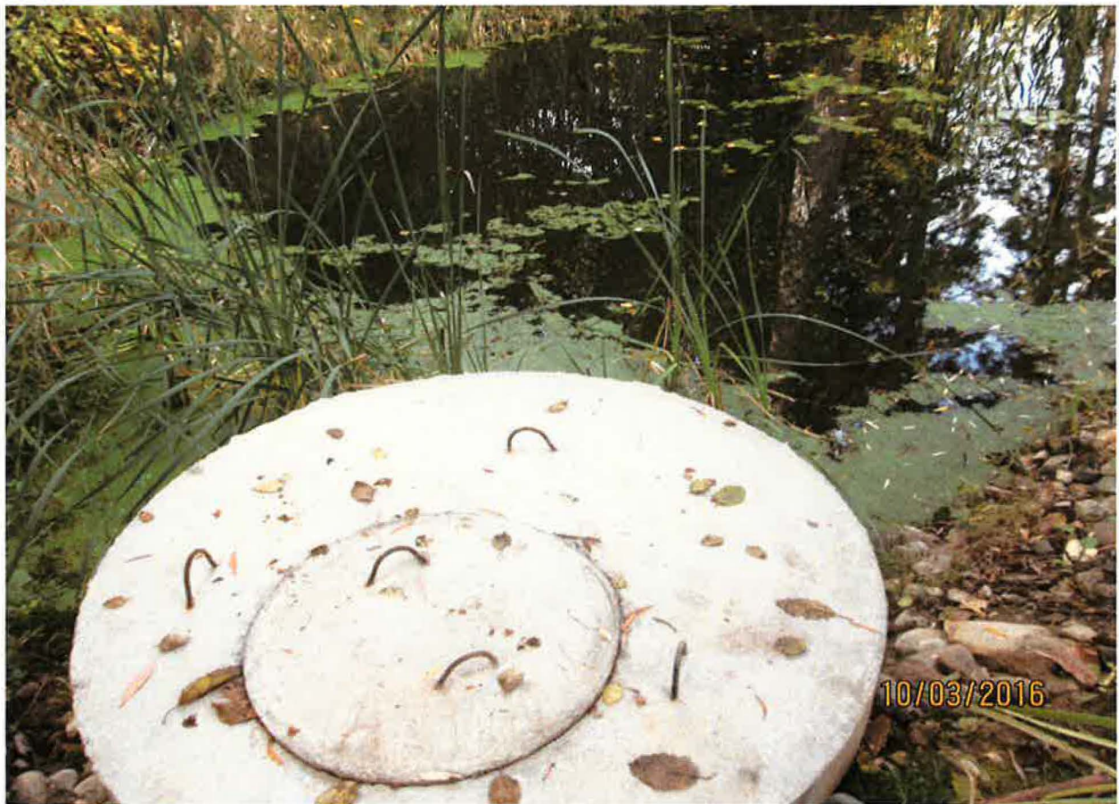
Culvert/ cistern in pond.
