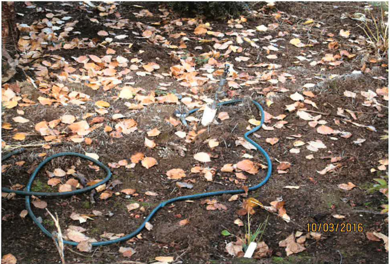
Sprinkler head with connection for hose.
