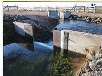
Old Curran Ranch 36-16948 November 14, 2019 Foreground: 2 ft. Standard Rectangular Contracted Weir Background: 18 inch buried pipe begins at old weir structure
