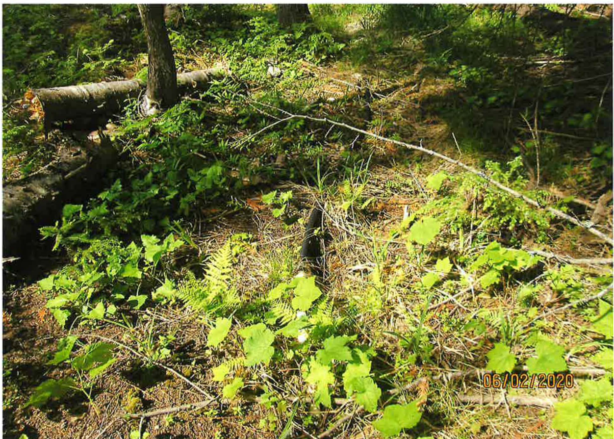
PVC PIPE WATER CONVEYANCE DOWN HILL TO POND
