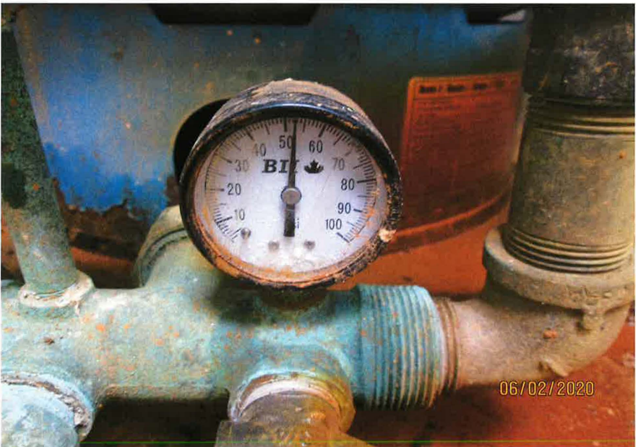
WATER SYSTEM OPERATING AT 52 PSI
