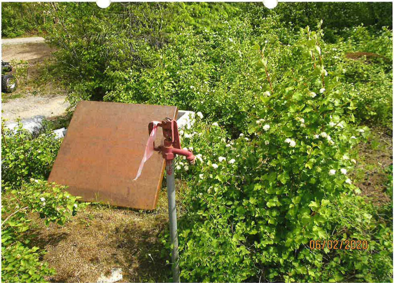
FIRE PROTECTION POU – FROST FREE HYDRANT
