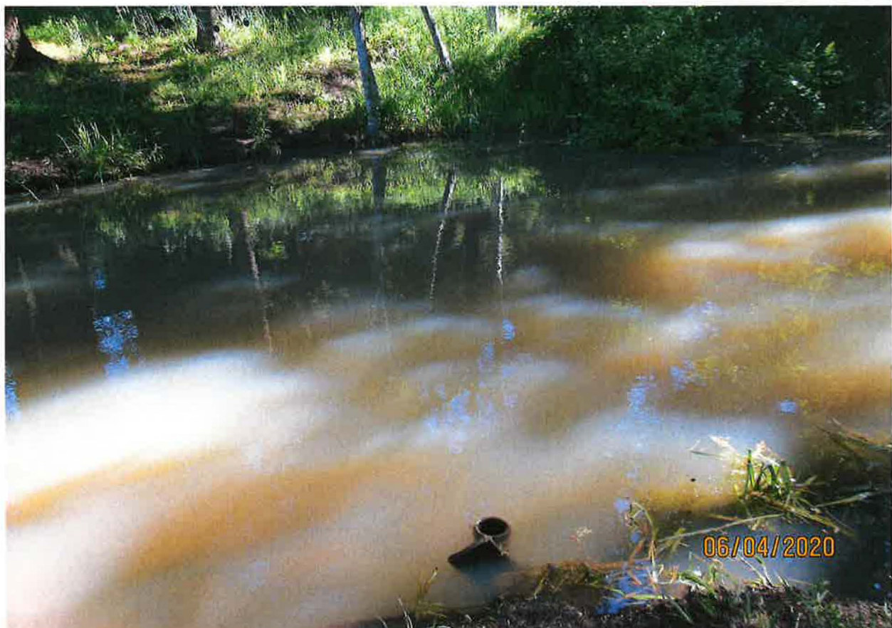
POND OVERFLOW PIPE
