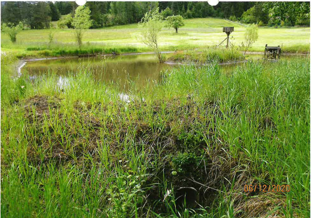
POD – POND 2 DAM
