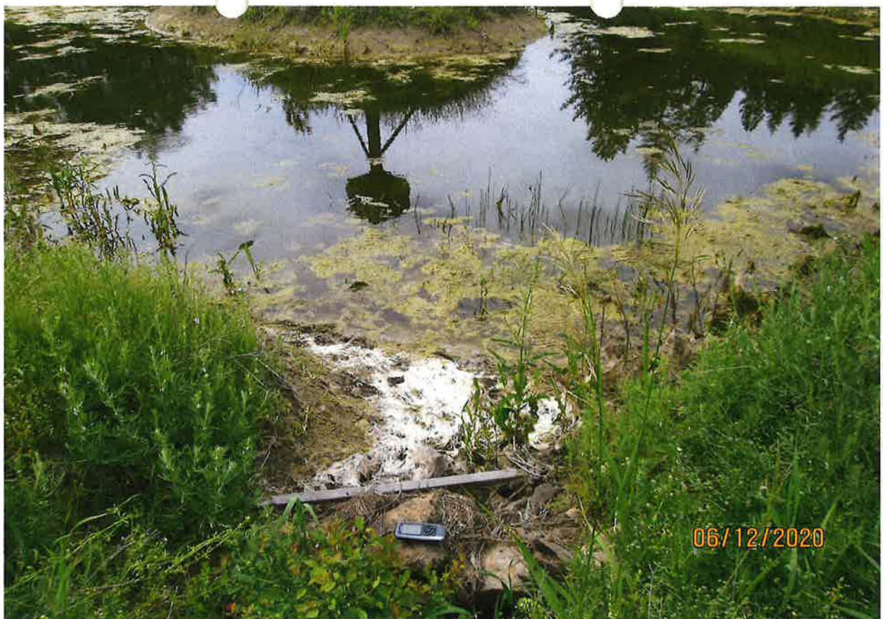
POD – POND 1 DAM
