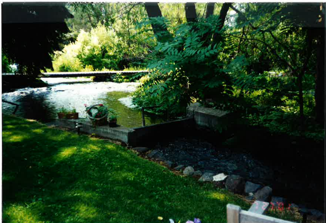
Diversion On Billingsley Cr. To Padgett Ditch
