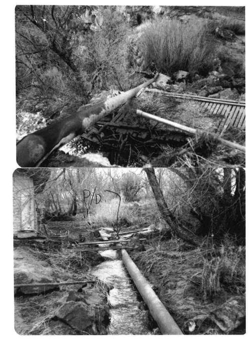
Penstock with converted pump used for therbite with generator.
