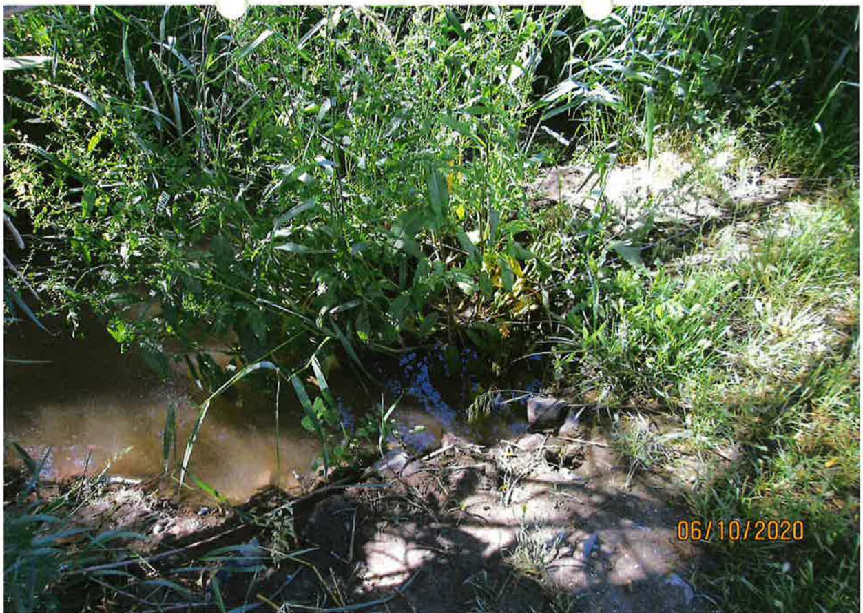
OUTFLOW FROM 24HR IMPOUNDMENT TO CREEK
