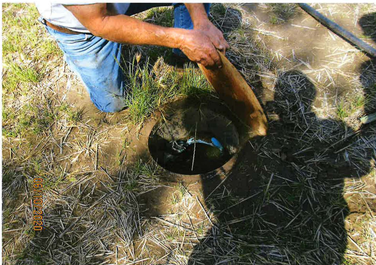
FLOW THROUGH PIPE FROM 24HR IMPOUNDMENT BACK TO CREEK
