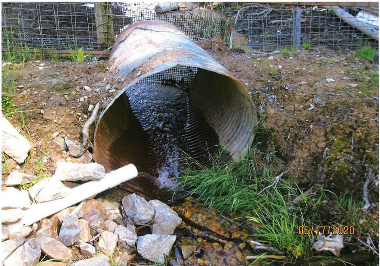
OVERFLOW FROM 1,000 GAL STORAGE TANK BACK TO CREEK
