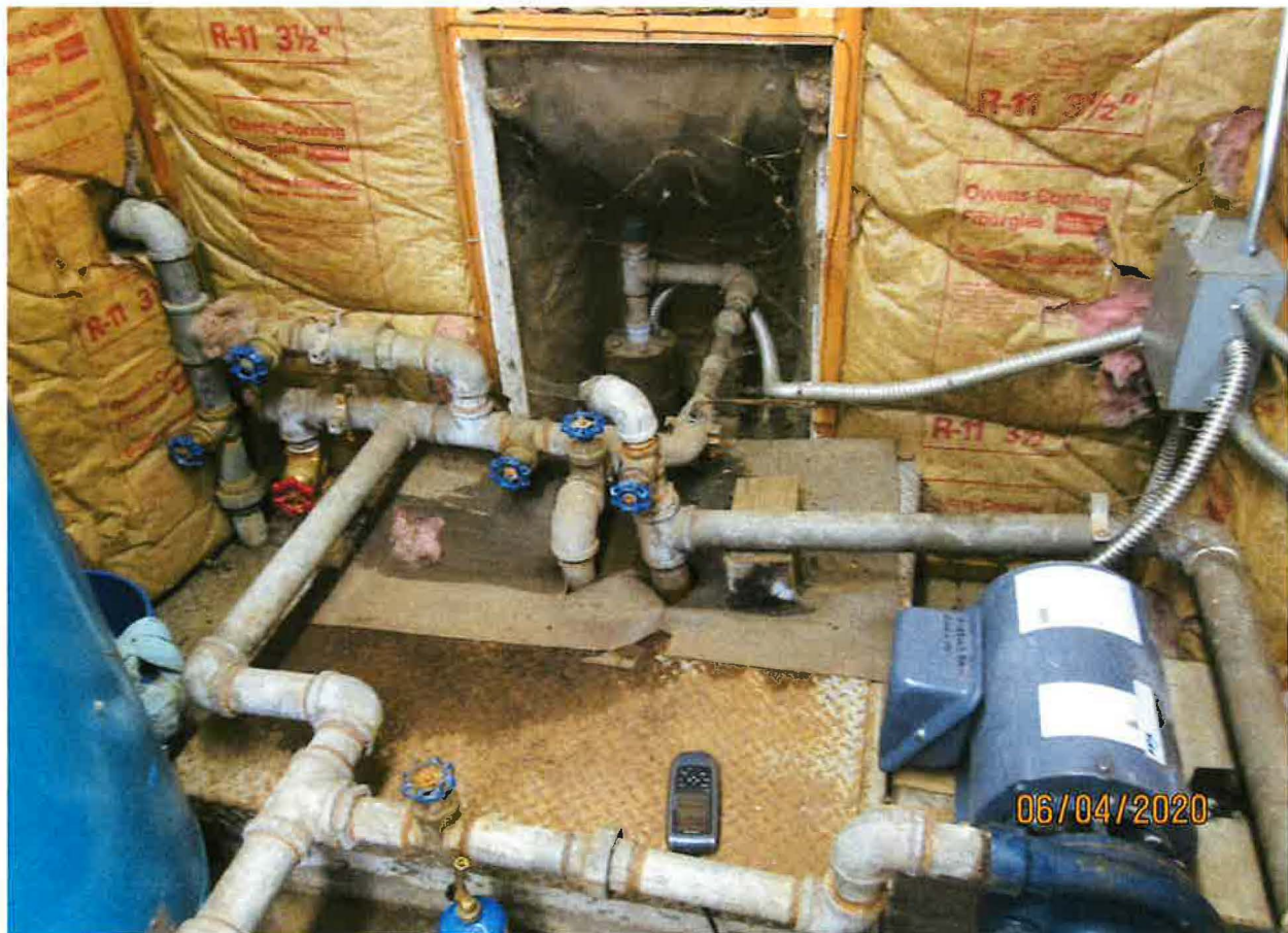
POD – WELL PERMIT No. 95-92-N-6
