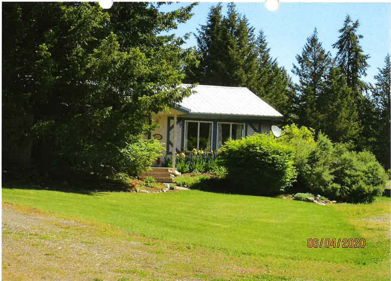
DOMESTIC / STOCKWATER POU – PINEGLEN WEST SUB, LT 1 BLK 1
