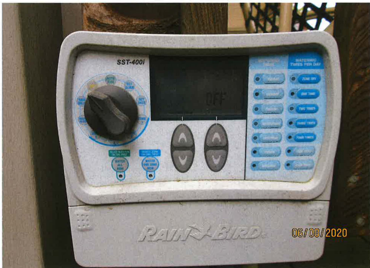
IRRIGATION SYSTEM AUTOMATIC SPRINKLER CONTROL
