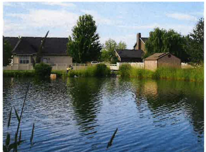
The gate for the southern outlet from the pond for excess surface water can be seen between the well (pumping water into the pond; IDWR staff removing flowmeter) and the pump house (southwest corner of the pond).
