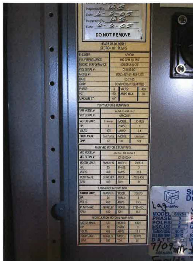
Labels for the motors and pumps within the well house
