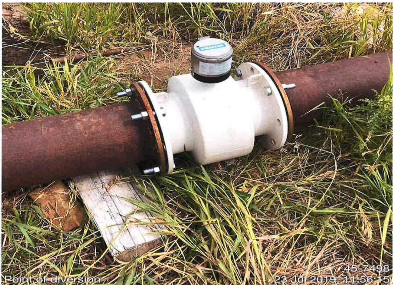
Meters Installed at each Pump
