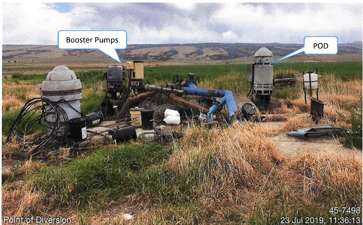
Above: Point of Diversion with Two Booster Pumps
