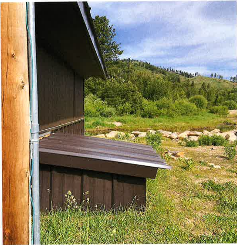
Fig. 3 – Well 2, right of pump house, view looking NW. GPS coordinates N 43.55458°, W 115.27505°.
