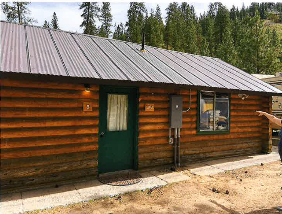
Fig. 14 – Laundry/Spa cabin adjacent to lodge. View looking north.
