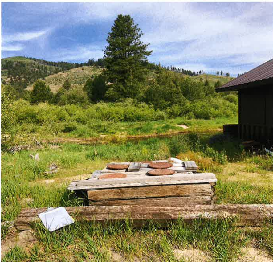
Fig. 2 – Well 1, left of pump house, view looking NW. GPS Coordinates N 43.55452°, W 115.27508°.
