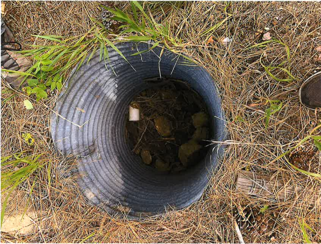
Fig. 7 – Culvert where domestic water source is stubbed in for residential lots.
