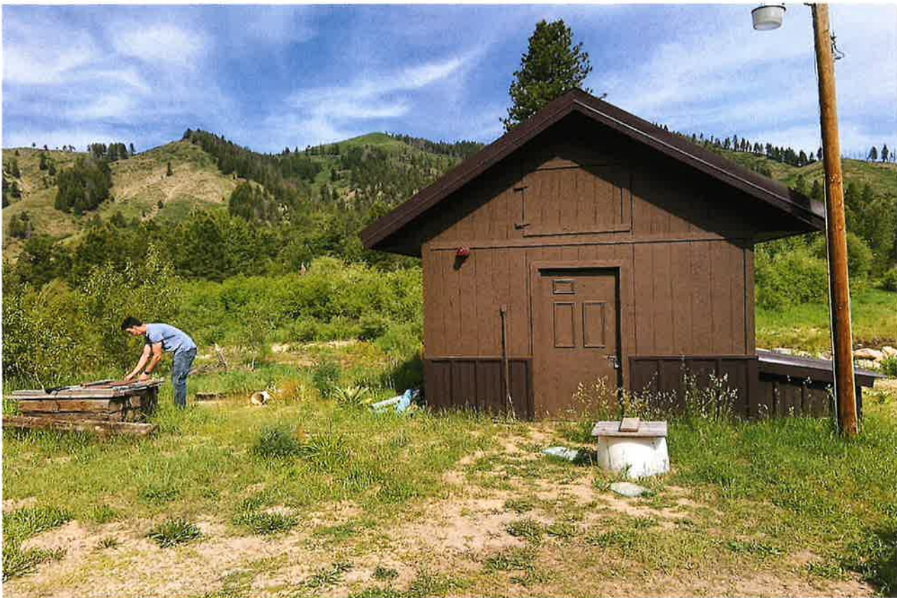
Fig. 1 – Pump house, Well 1 left of pump house, Well 2 right of pump house. View looking NW.
