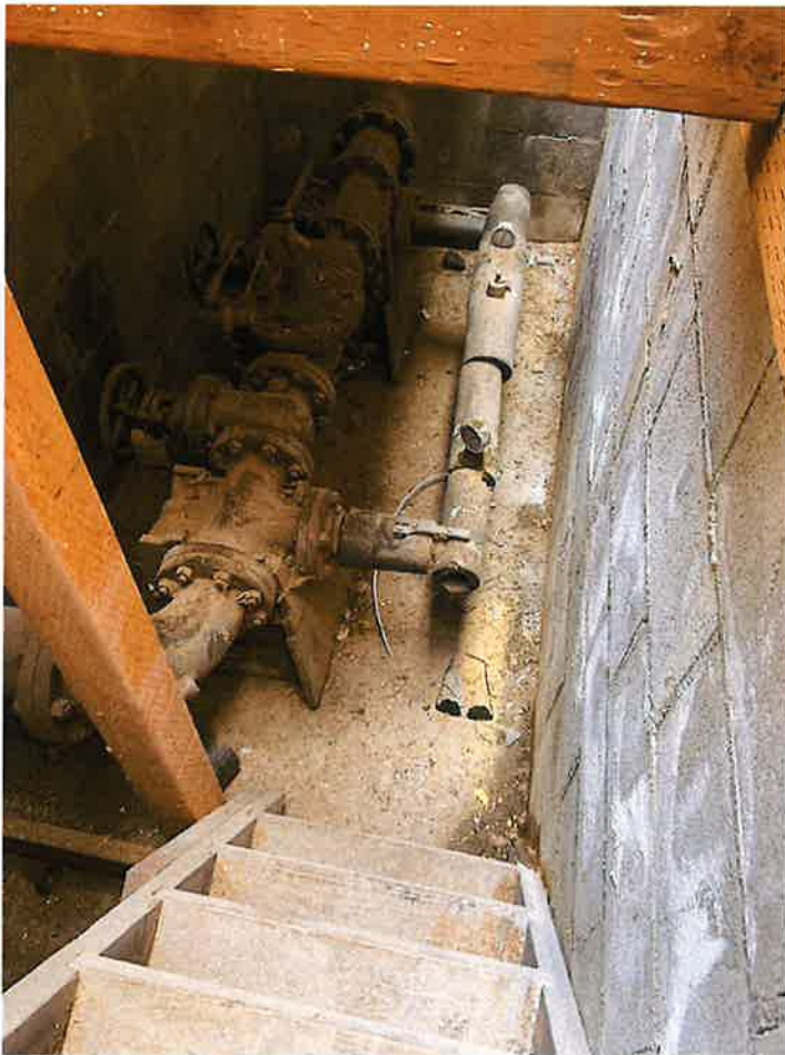
Fig. 10 – Pressure reduction system. Sunglasses for scale.
