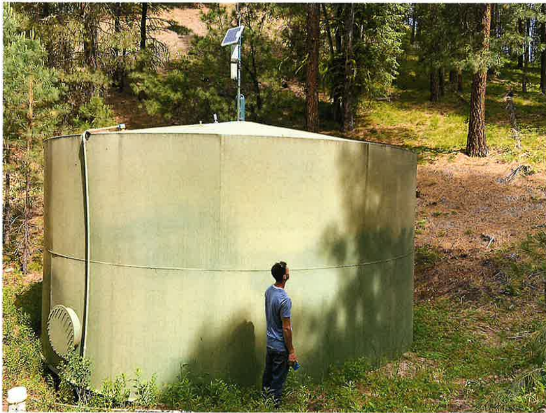
Fig. 11 – Holding tank, approx. 12' tall, 25-30' diameter. WRS Patrick Kelly for scale.
