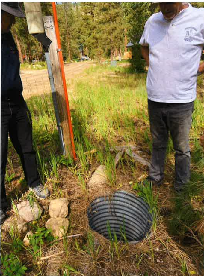
Fig. 8 – Culvert in a residential lot currently being developed in the Willis Carries Paradise Subdivision.
