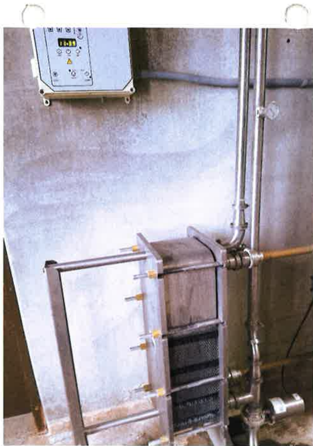
Looking at plate cooler (water is reused).
