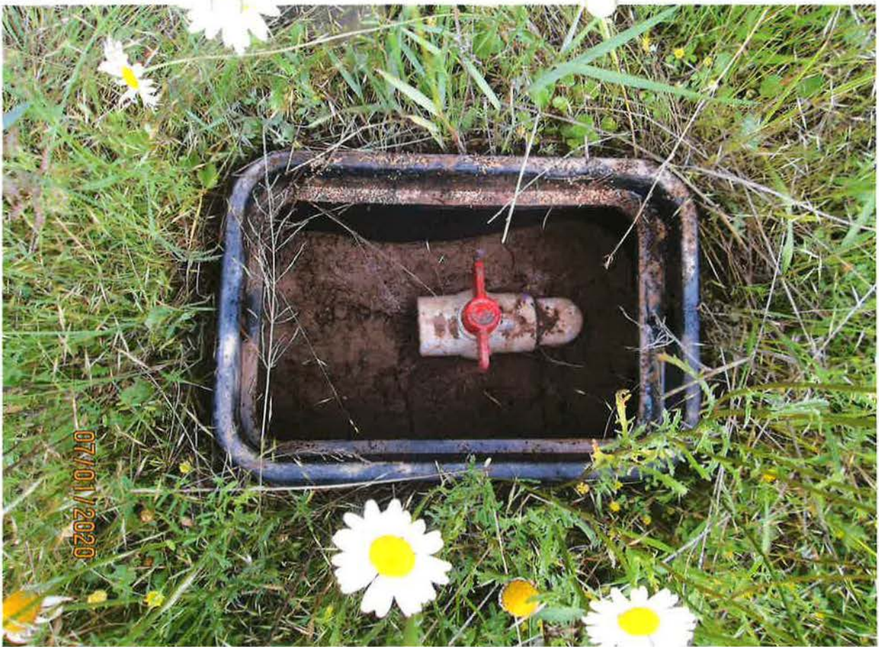
IRRIGATION SYSTEM RISES OFF BURIED MAIN LINE
