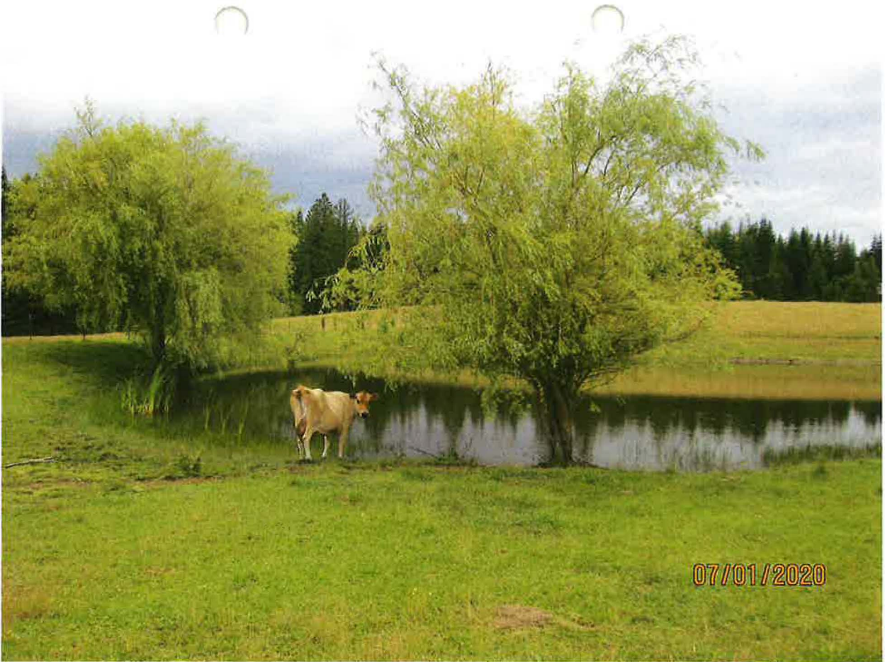
POD – POND 2 DAM, STOCKWATER FROM STORAGE POU
