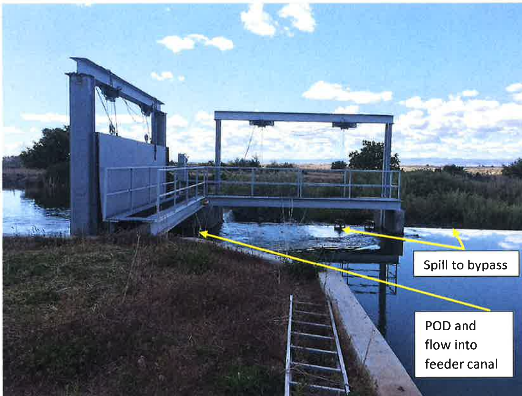
Photo 4a ABOVE: Point of Diversion for Permit 37-21297, and spill to bypass (Little Wood River).
