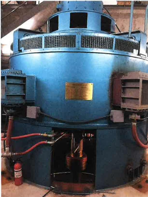
Photo 4c LEFT: Turbine & generator set with fixed shaft.
