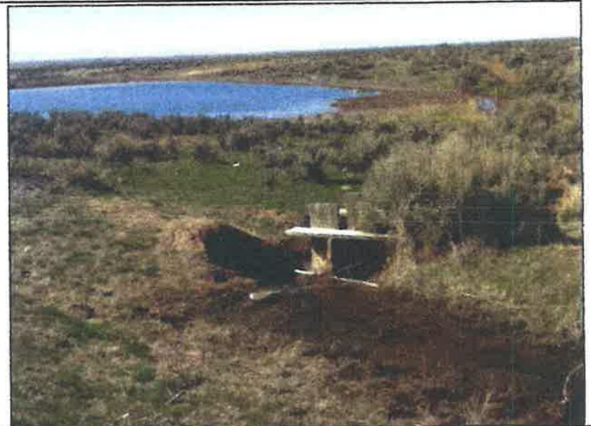
3-13-2014 photograph looking southwest past the washed out diversion structure on the 4-Mile Ditch to the full CDN Upper Ryegrass reservoir in the background. Washout points to higher earlier flows.
