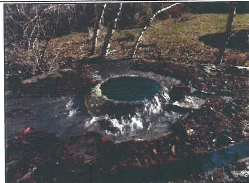
3-13-2014 Cold Springs Creek water entering the CDN bubbler and flowing out on to a trash screen which separates leaves, debris, and the many small fish seen stranded on the screen.
