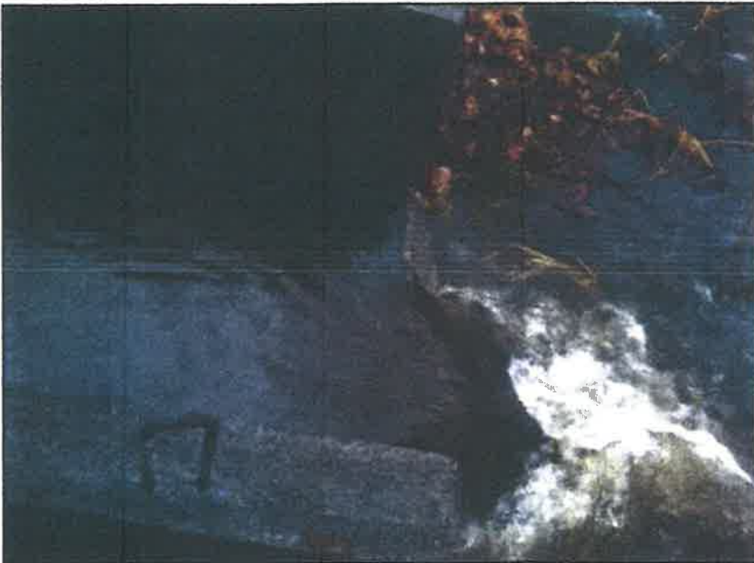
2-14-2014 Casa Del Norte's Elk Pen/Four-Mile Ditch weir. An estimated 2,700 gallons per minute was passing through weir and 450 gpm was bypassing it. Weir plate in concrete raceway is over-flooded.
