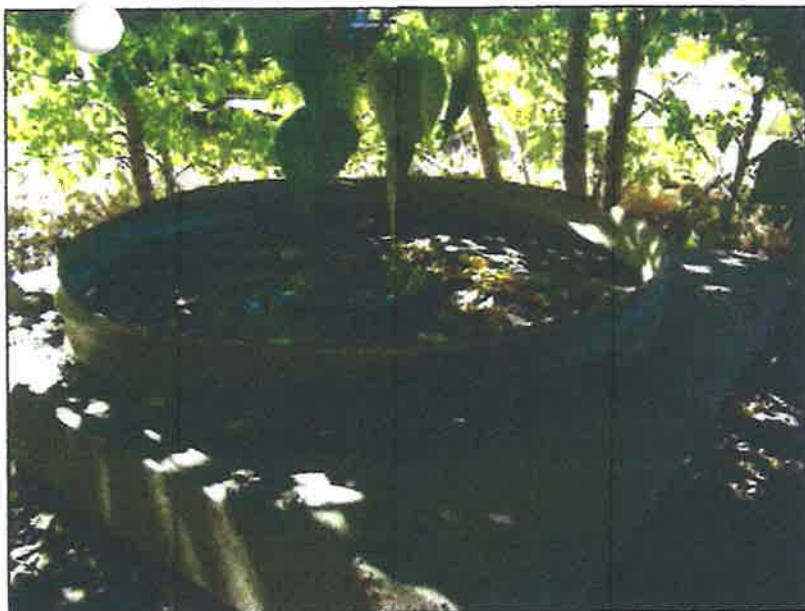
7-22-2013 photo of CDN's "bubbler", a trash screen to separate debris from the stream intake prior to water entering a pipe to the irrigation distribution system. Water enters via vertical pipe at center. Corrugated steel ring raises the water level (head) to drive more water through.
