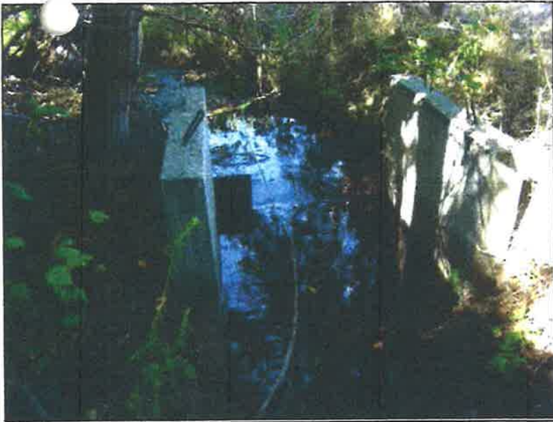
7-22-2013 photograph of the measurement weir for the Elk Pen Ditch just below the CDN's Upper Main Cold Springs Creek Diversion with only a few tens of gallons per minute flowing over the weir plate.
