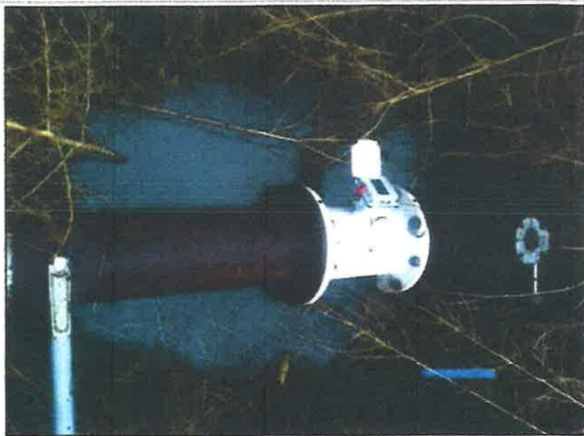
2-14-2014 CDN #4 Pivot/Reservoir flow-meter. This is the third site visit where the flow-meter was found to be inoperative and/or inaccurately showing the current flow.
