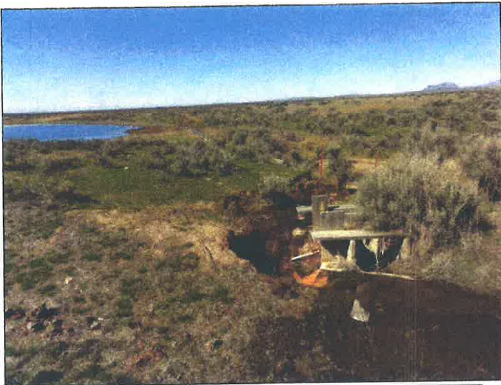
3-13-2014 photograph looking southwest past the washed out diversion structure on the 4-Mile Ditch to the CDN Upper Ryegrass reservoir in the background. Washout points to higher earlier flows.
