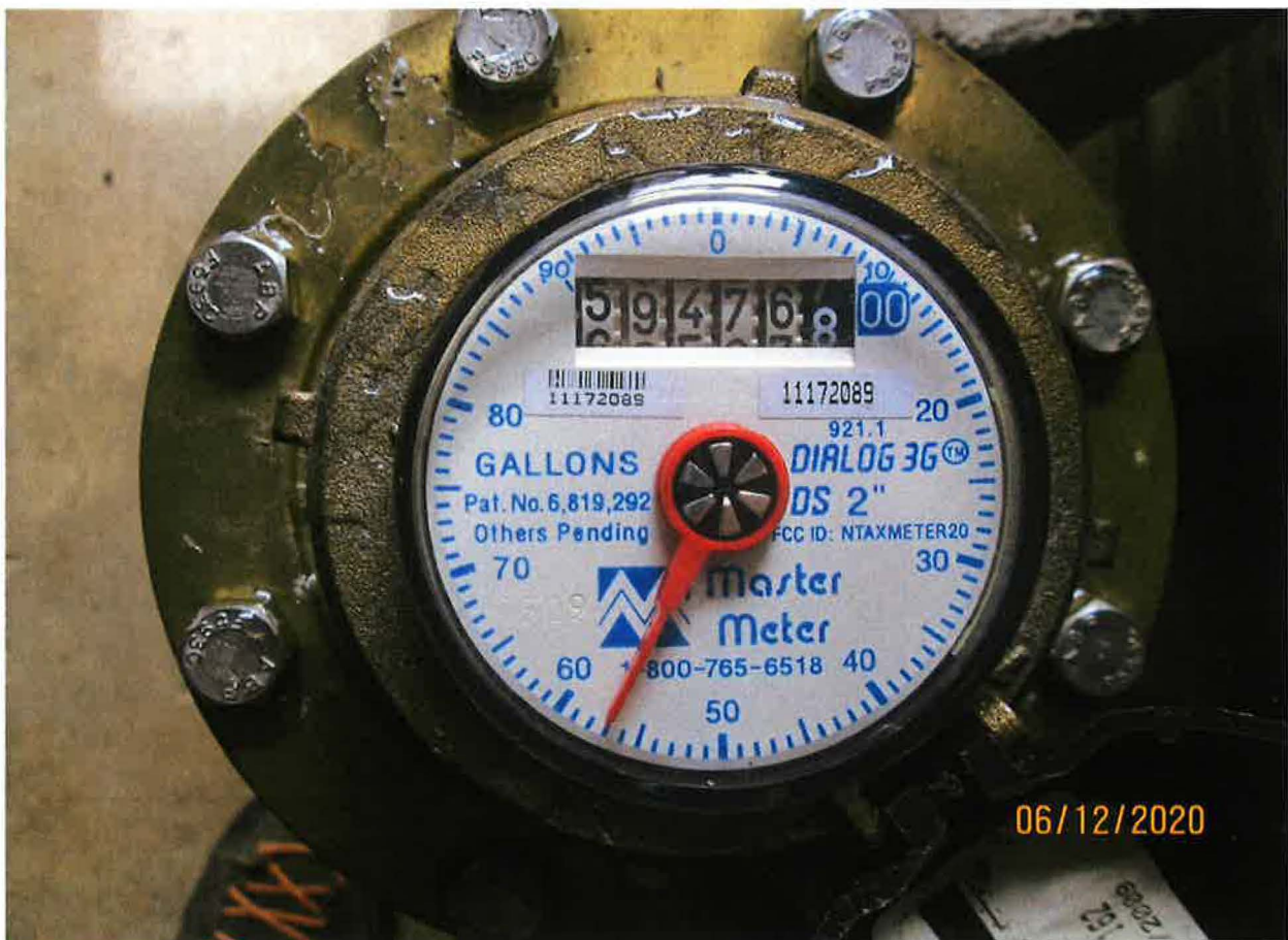
WATER METER IN PUMP HOUSE
