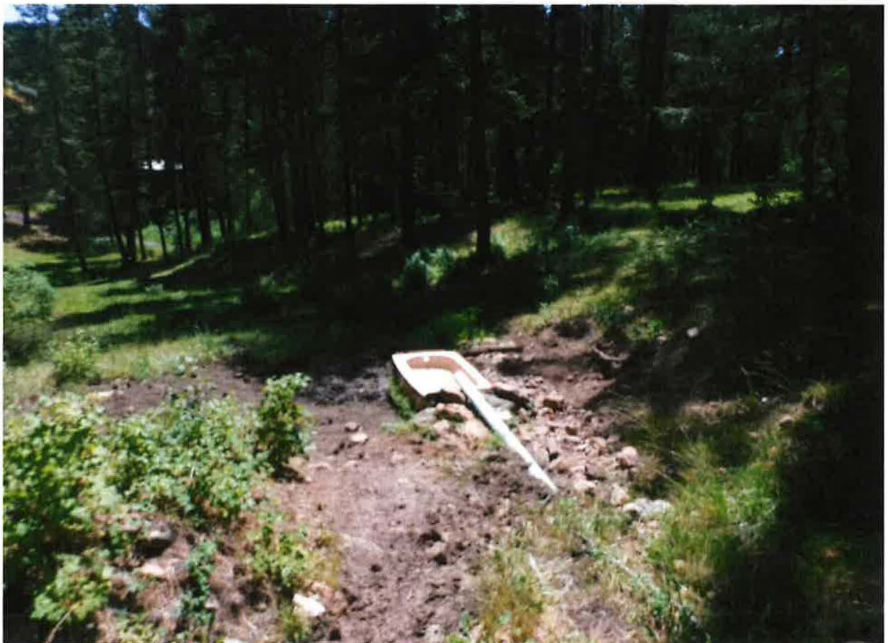
POD – 6" STORM PIPE TO BURIED SPRING BOX
