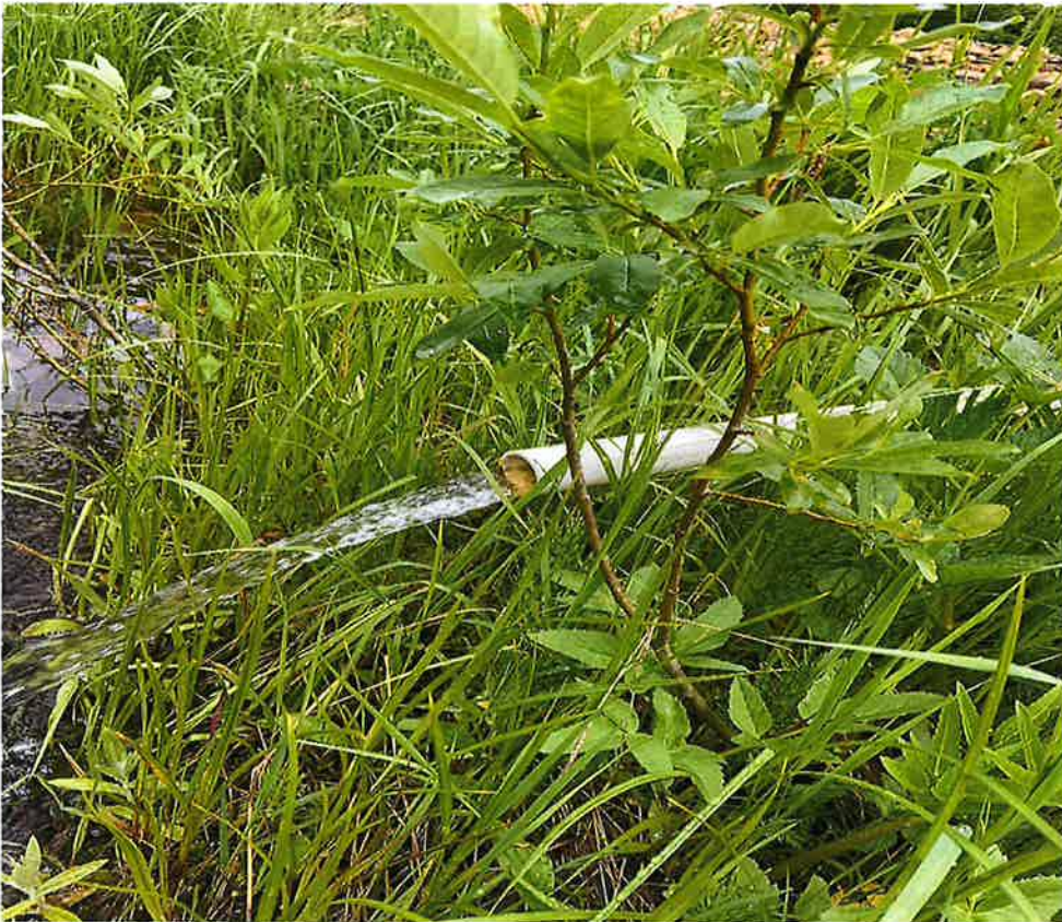
Fig. 7 – Close-up of discharge of overflow into Crooked Creek after heavy rains.
