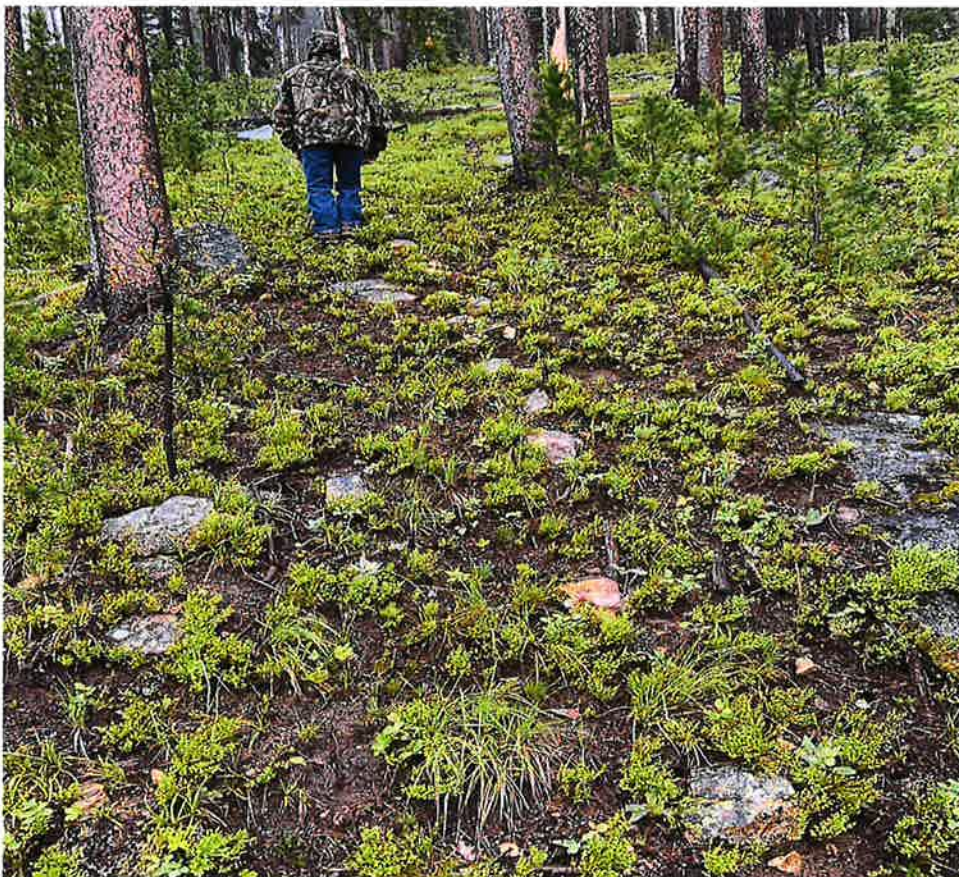
Fig. 2 – Rock line indicating path of buried 1.25" pvc pipe from spring to storage tanks
