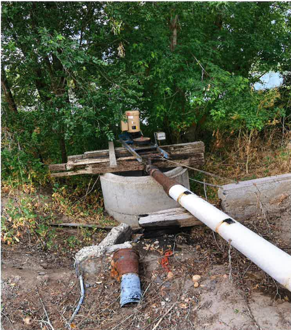
Fig. 2 – Pump with PVC line coming out bringing water to the bubbler.
