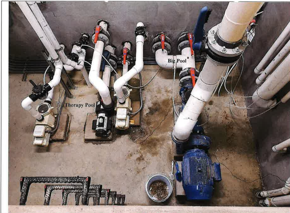
Pumps used to circulate water in each pool.
