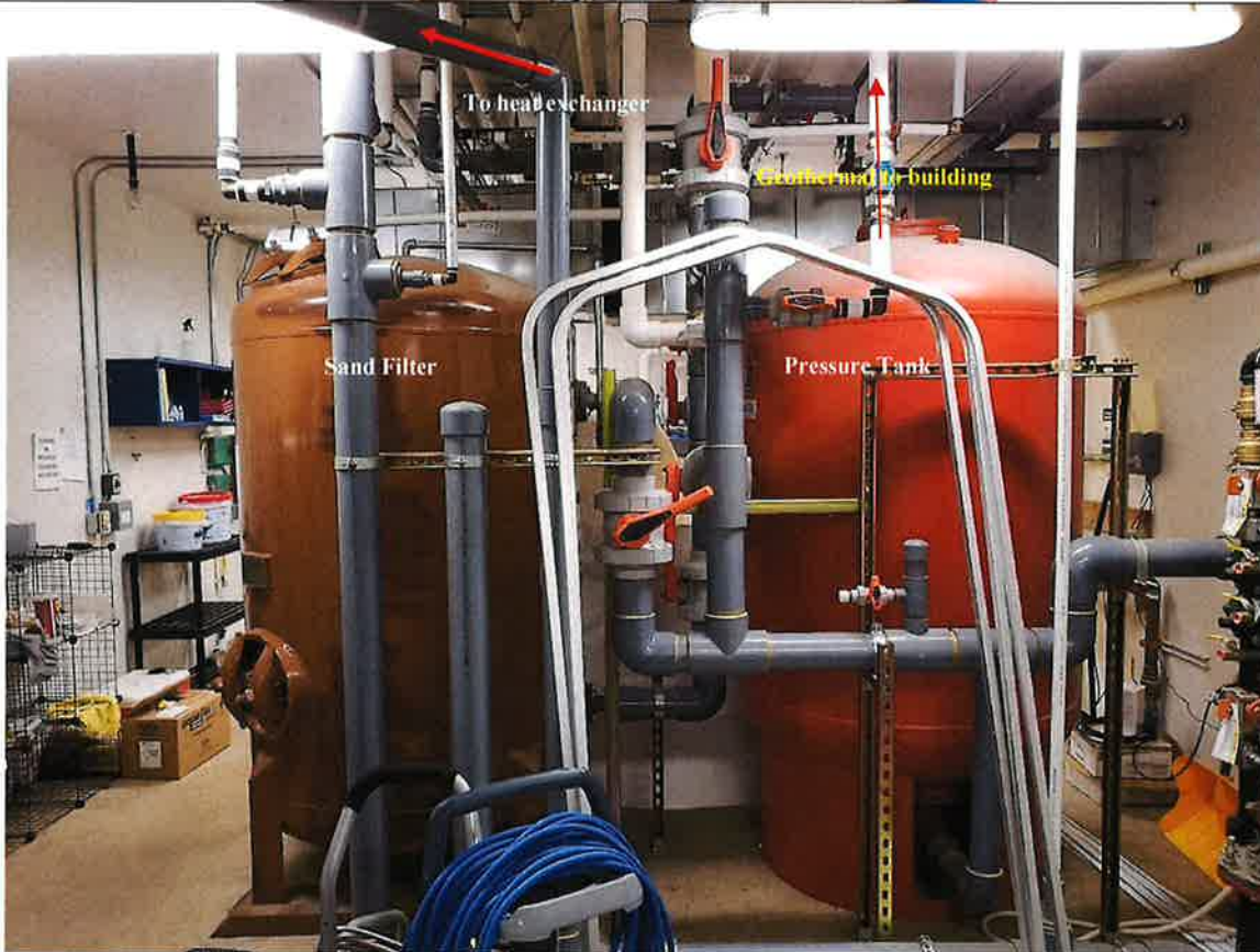
Geothermal water is ran through a pressure tank and/or sand filter before being used.
