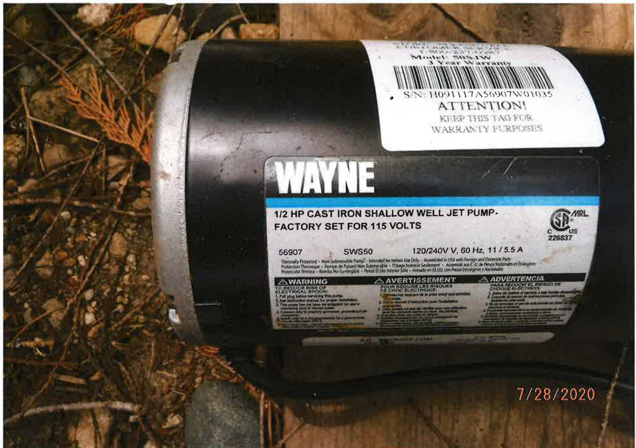
½ HP WATER TRANSFER PUMP AT POD
