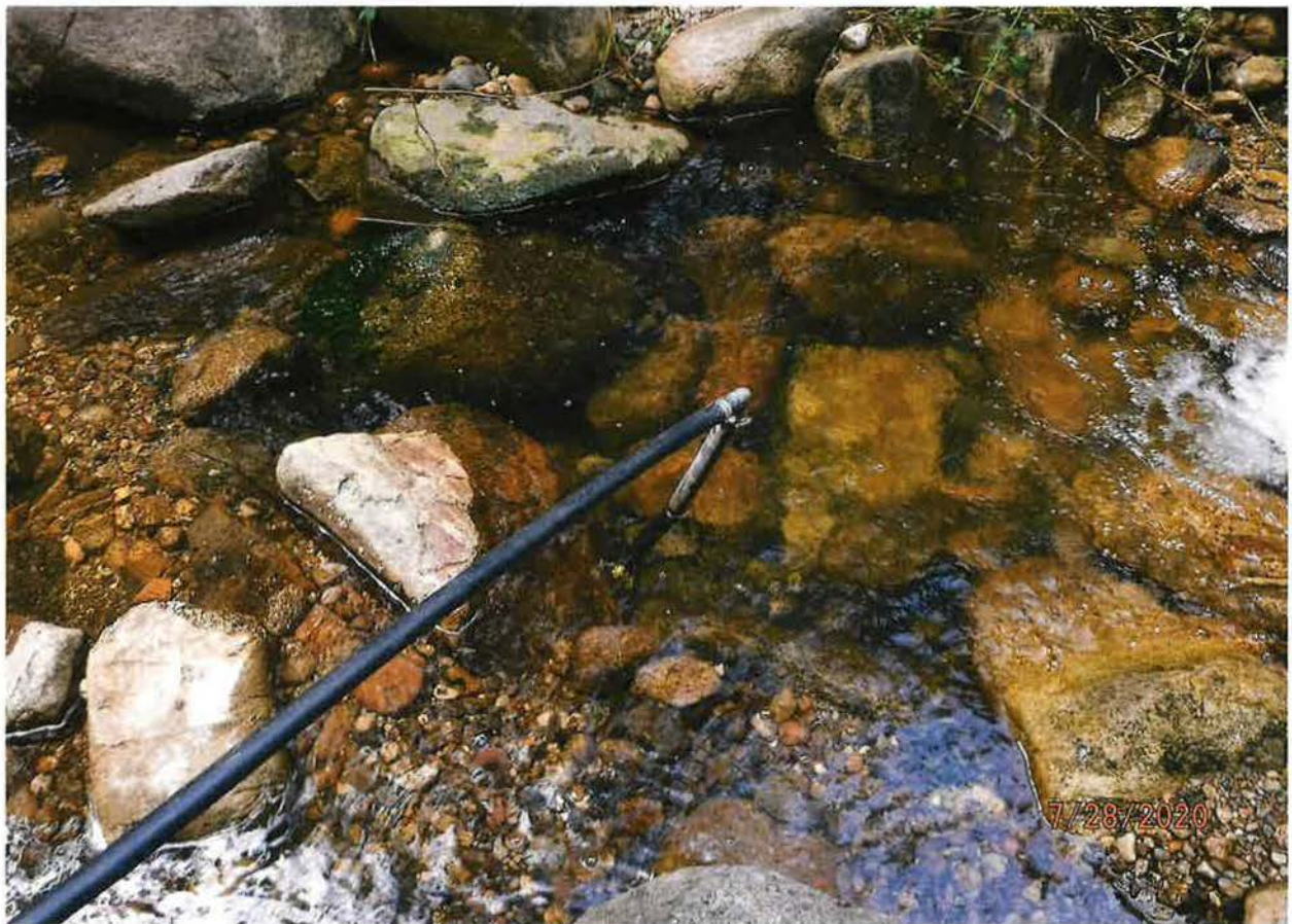
POD – SCREENED PVC PIPE IN CREEK
