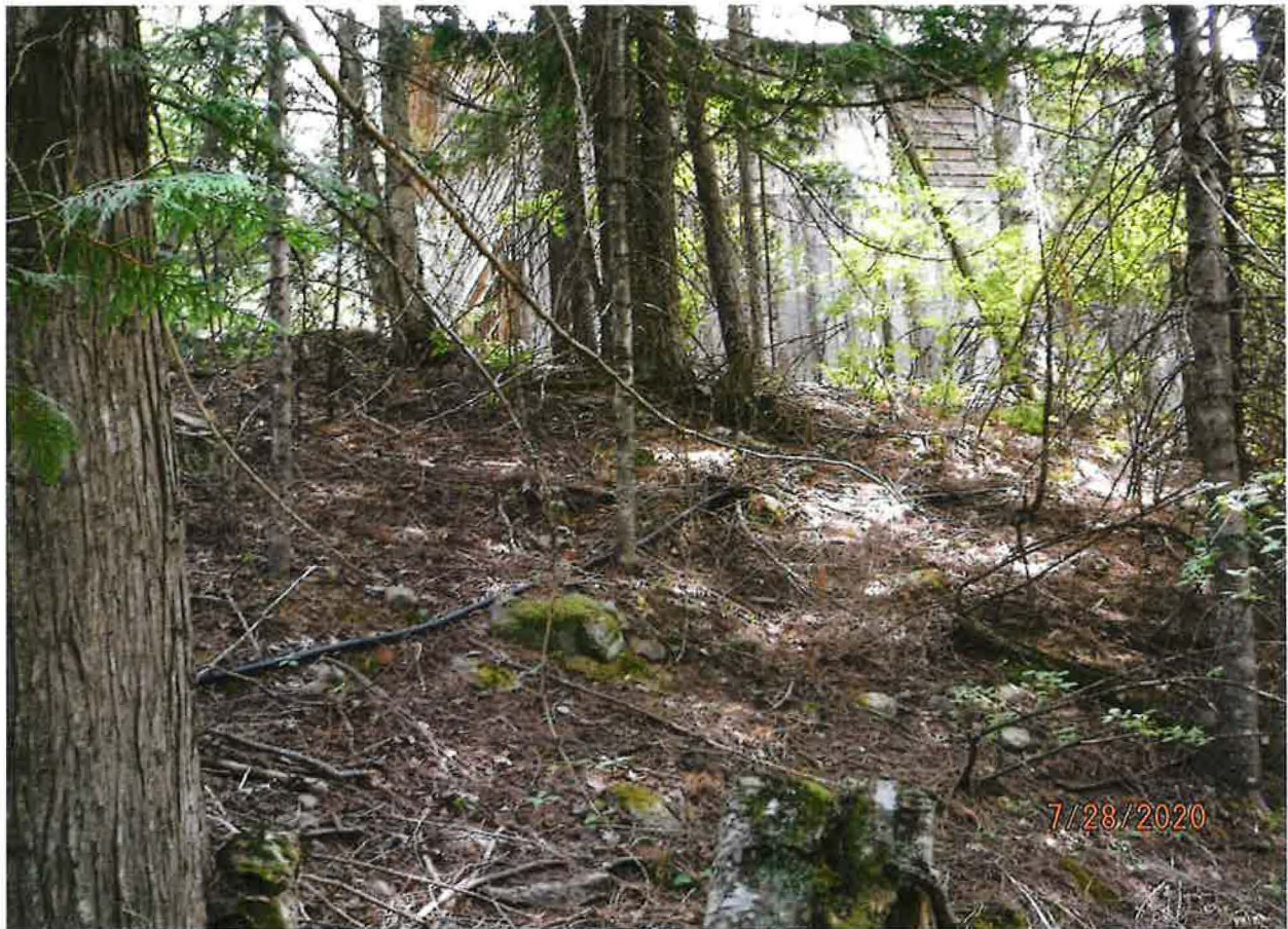
2" PVC PIPE UPHILL FROM POD TO POU
