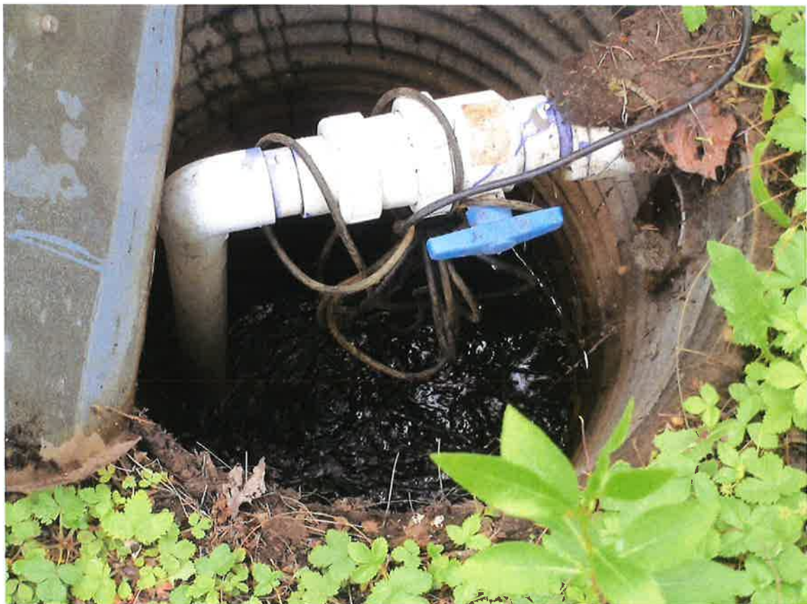
Sump – Submerged pump lifts water approximately 3' to head of stream.
