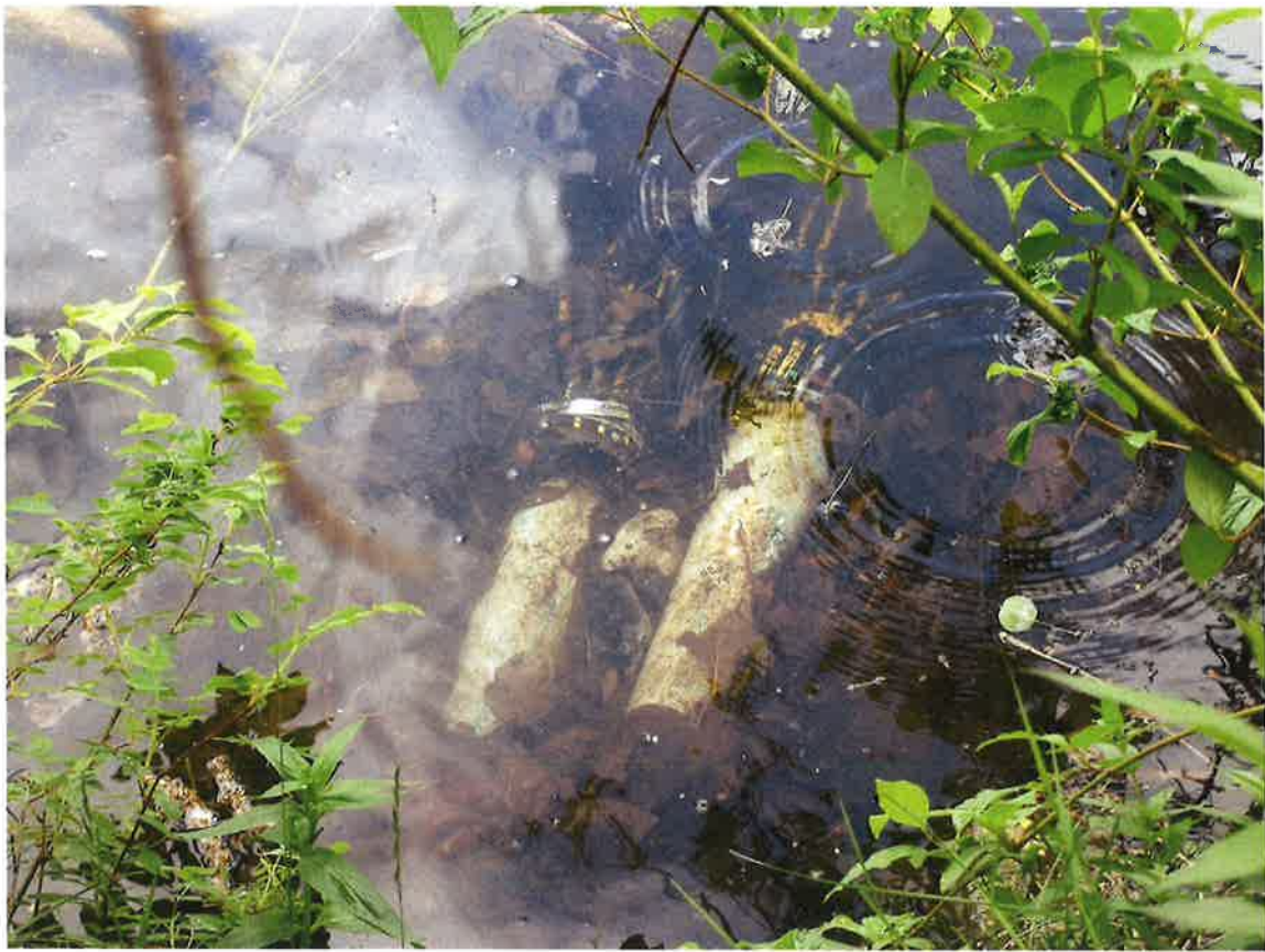
POD – Two 3" diameter PVC pipes carry water by gravity from large pond to sump.
