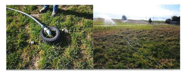
The above photos show the spigot at the first distribution point located closest to the well, and the irrigation hose which connects to the 4-way splitters.
