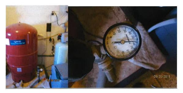
The above photos show the pump's pressure gauge, located adjacent to the home's precharge (red) tank.
