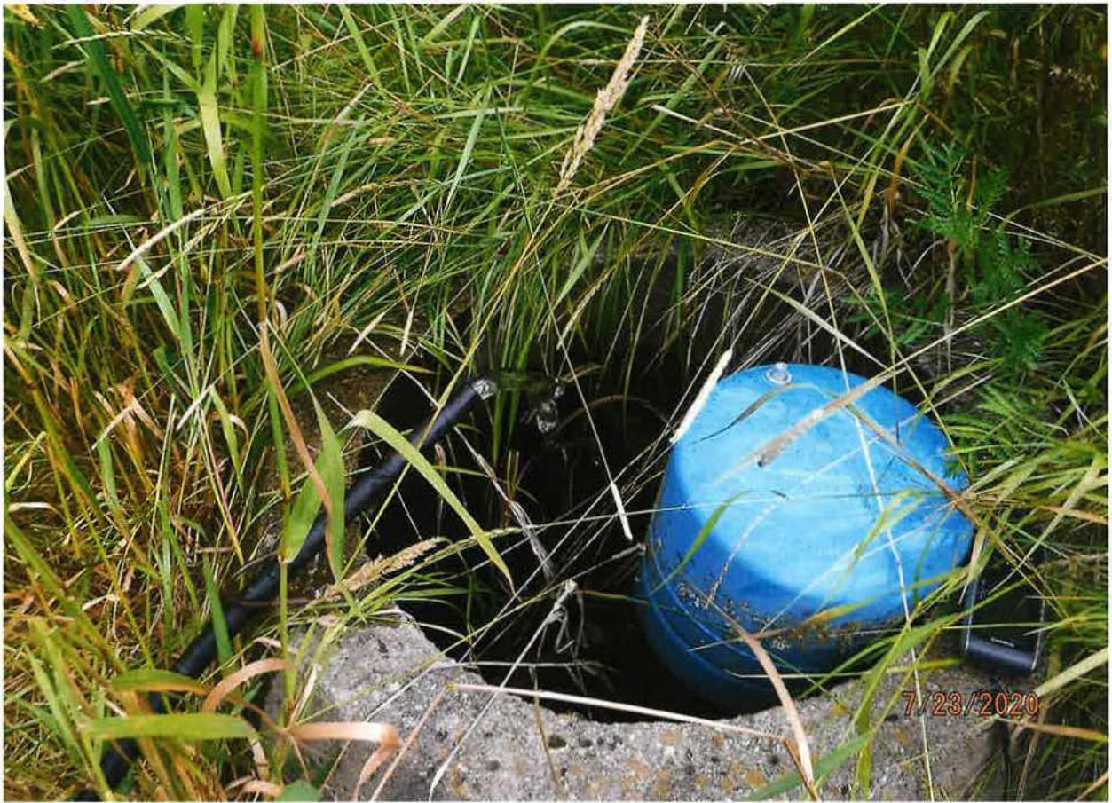
STORAGE CISTERN – 24 HOURS USE FOR IRRIGATION
