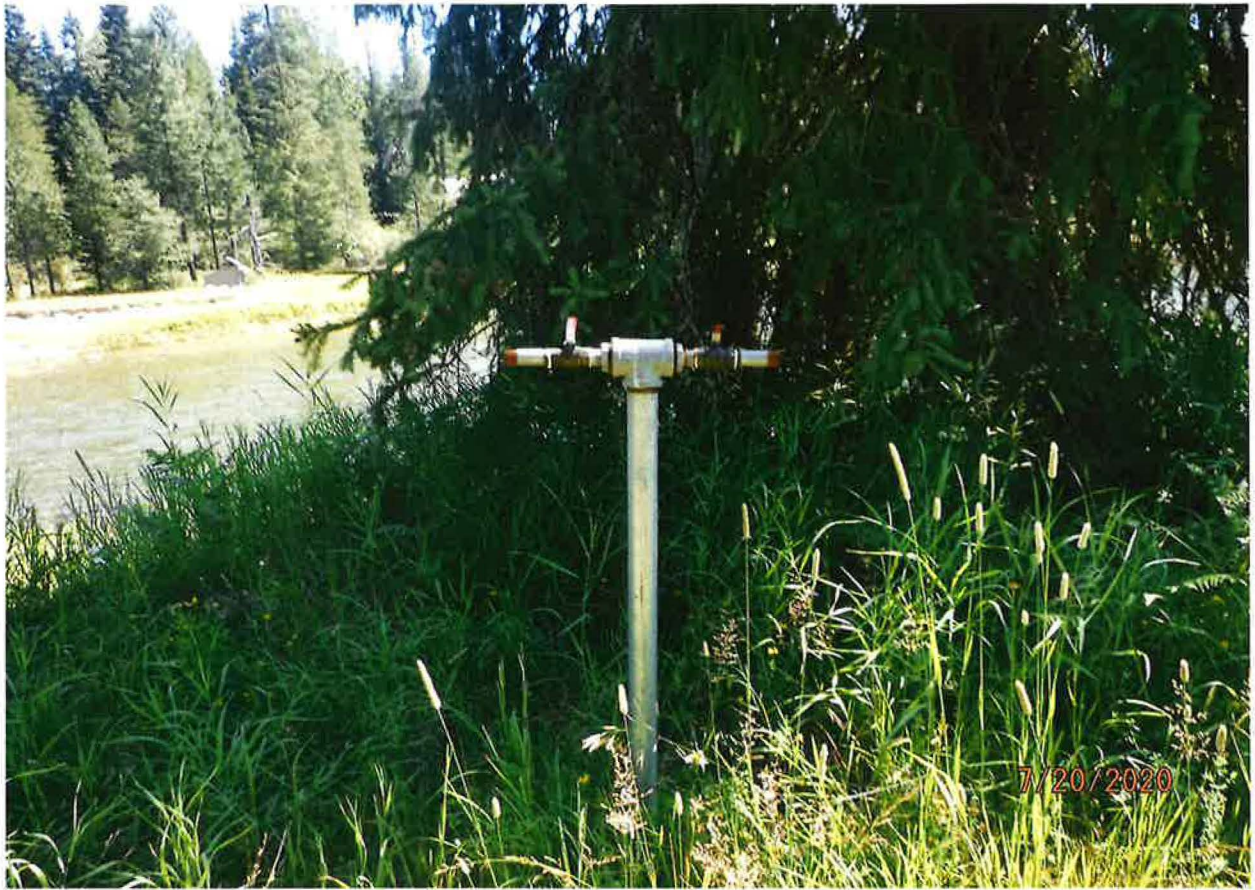
IRRIGATION RISERS OFF MAIN TRUNK PIPE LINE
