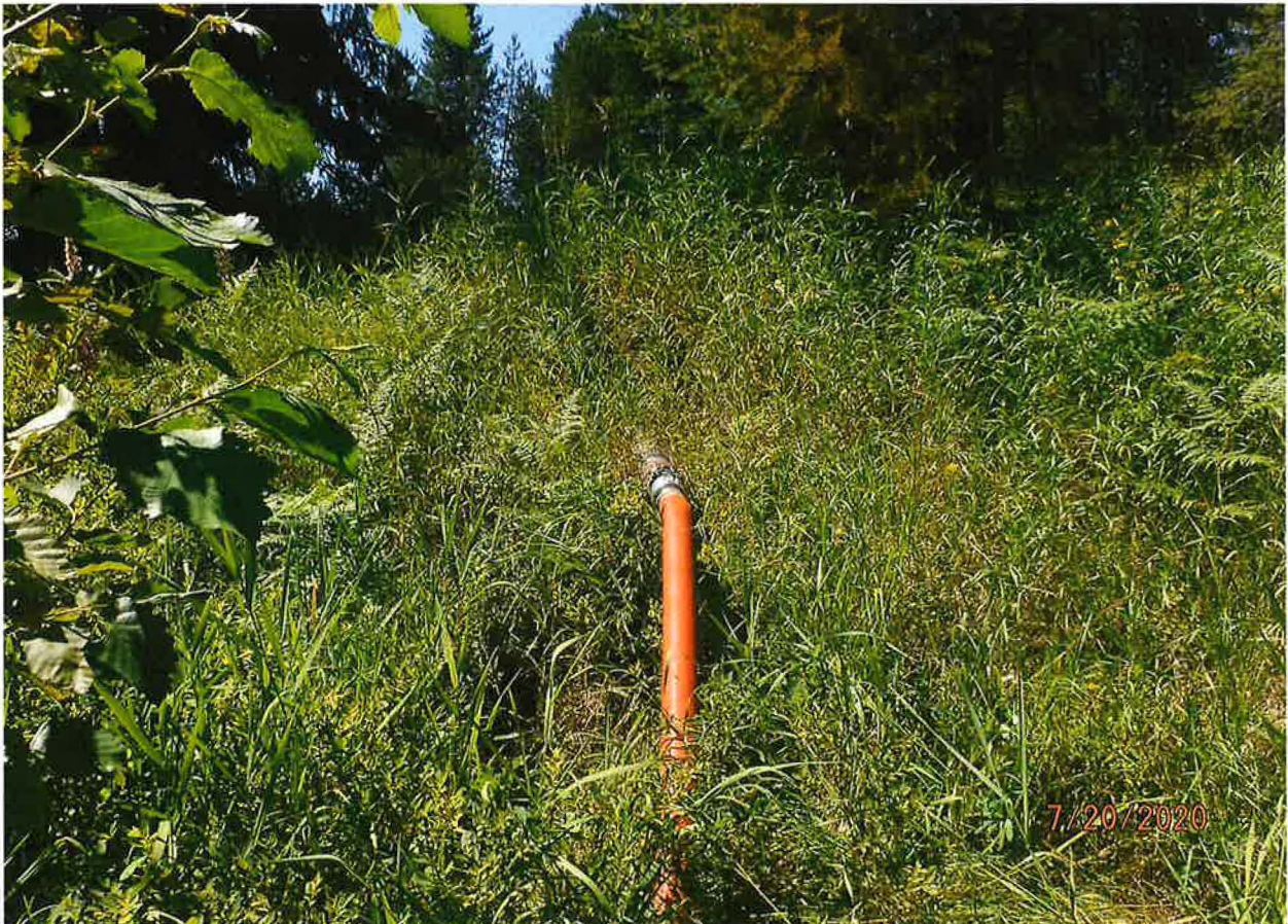
FLEX PIPE FROM POD TO IRRIGATION MAIN TRUNK LINE
