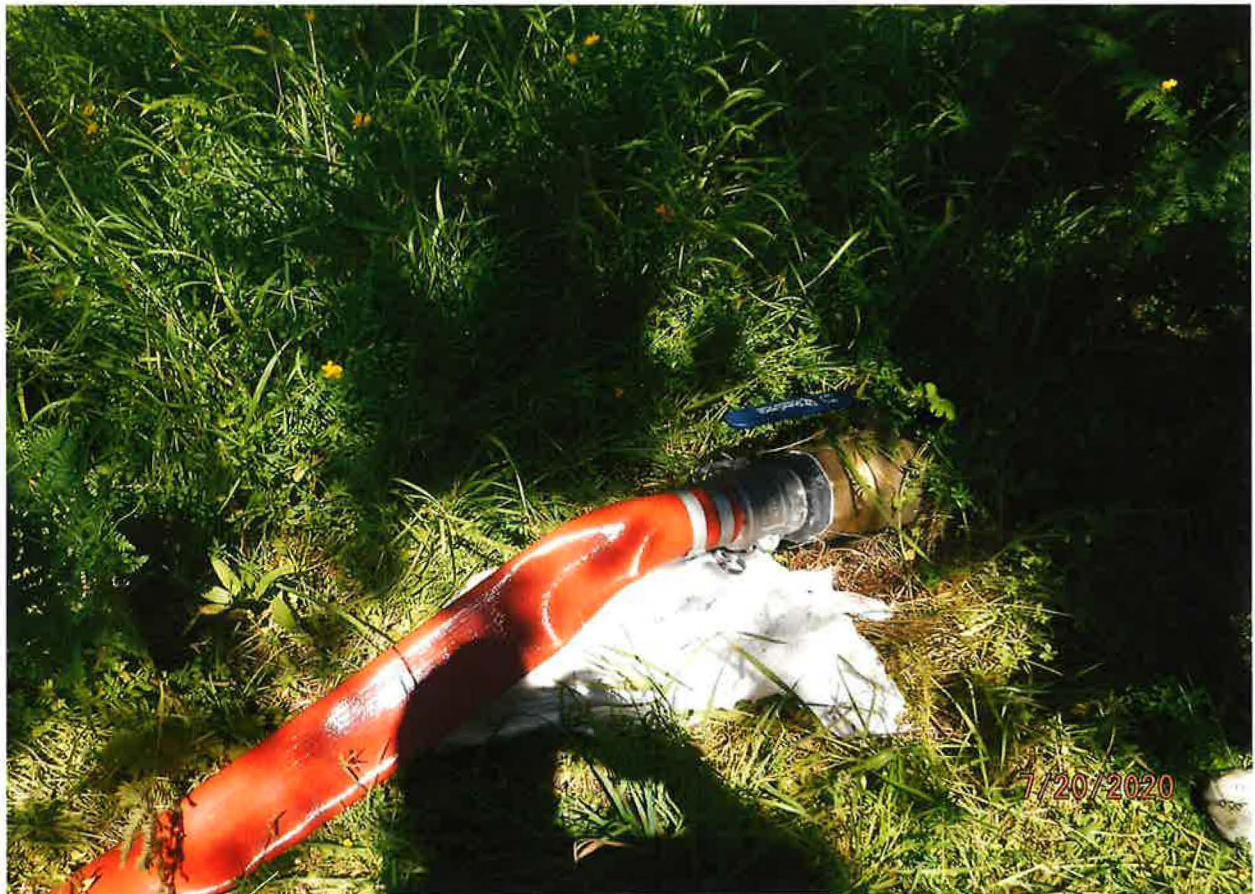
IRRIGATION PIPE FROM MAIN TRUNK LINE TO SPRINKLER SYSTEM
