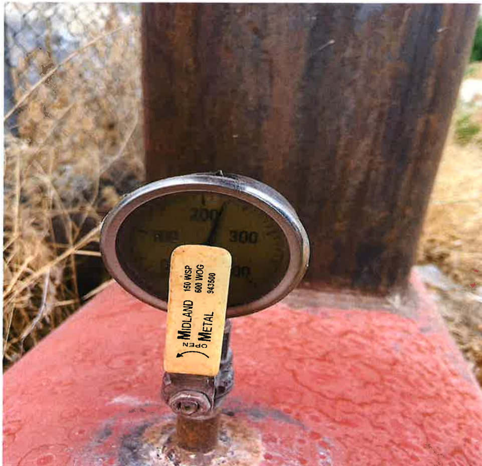
Fig. 4 – Pressure gauge reading ~225 psi where both pump flows meet into one pipe.
