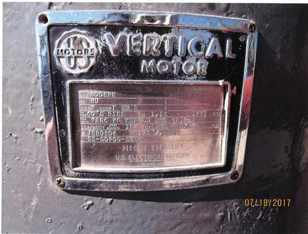
Figure 6. Motor tag on one of the pump housings at the pumping station.
