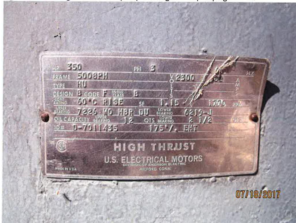
Figure 7. Motor tag on the other pump housing at the POD pumping station.
