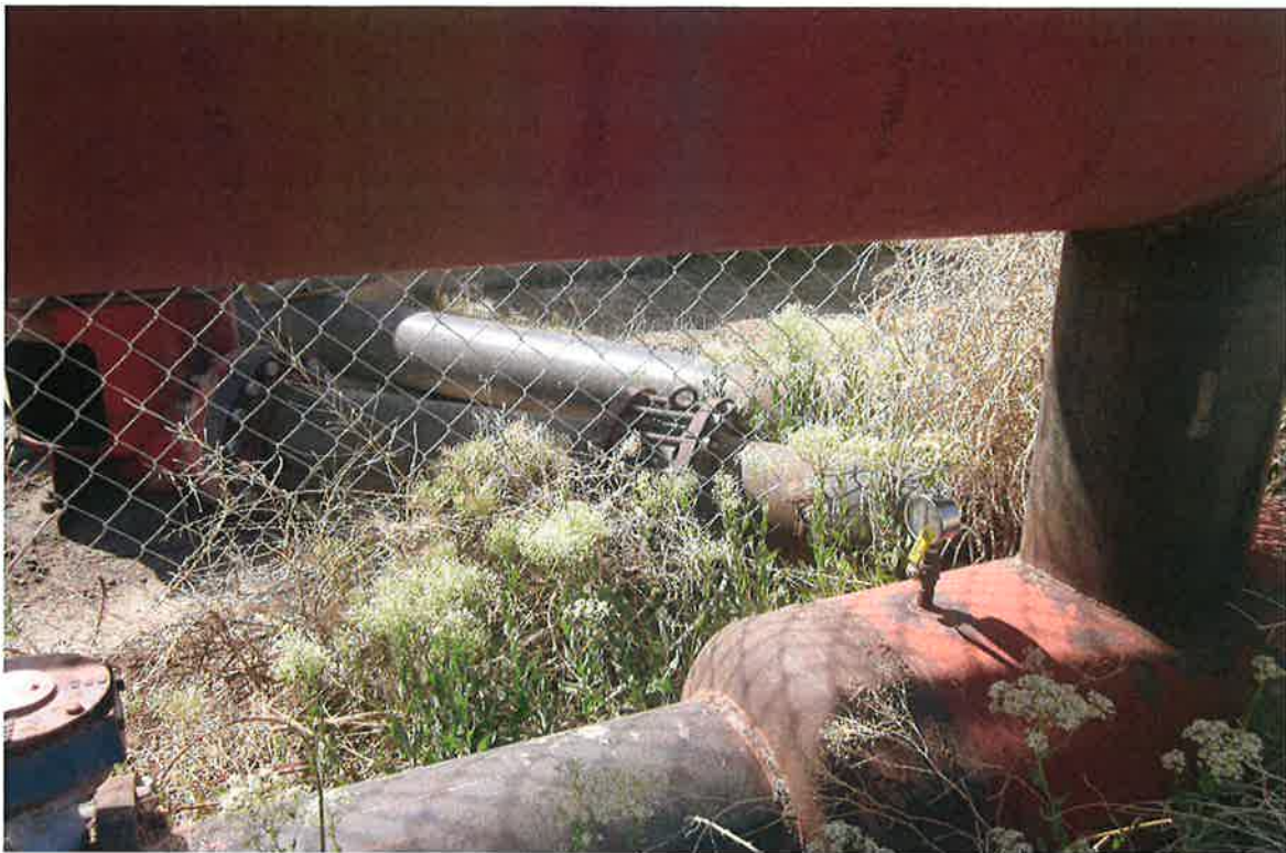
Pressure gauge – reading was 200 psi during exam, with one turbine operating. The 12" diameter piping from the turbines seen center.
