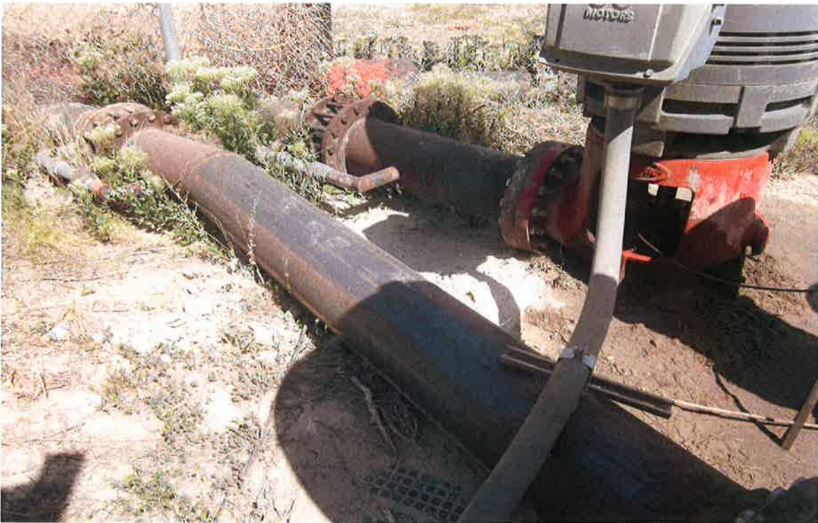
Another view of the 12" diameter piping from the turbines to the 18" diameter steel pipe.
