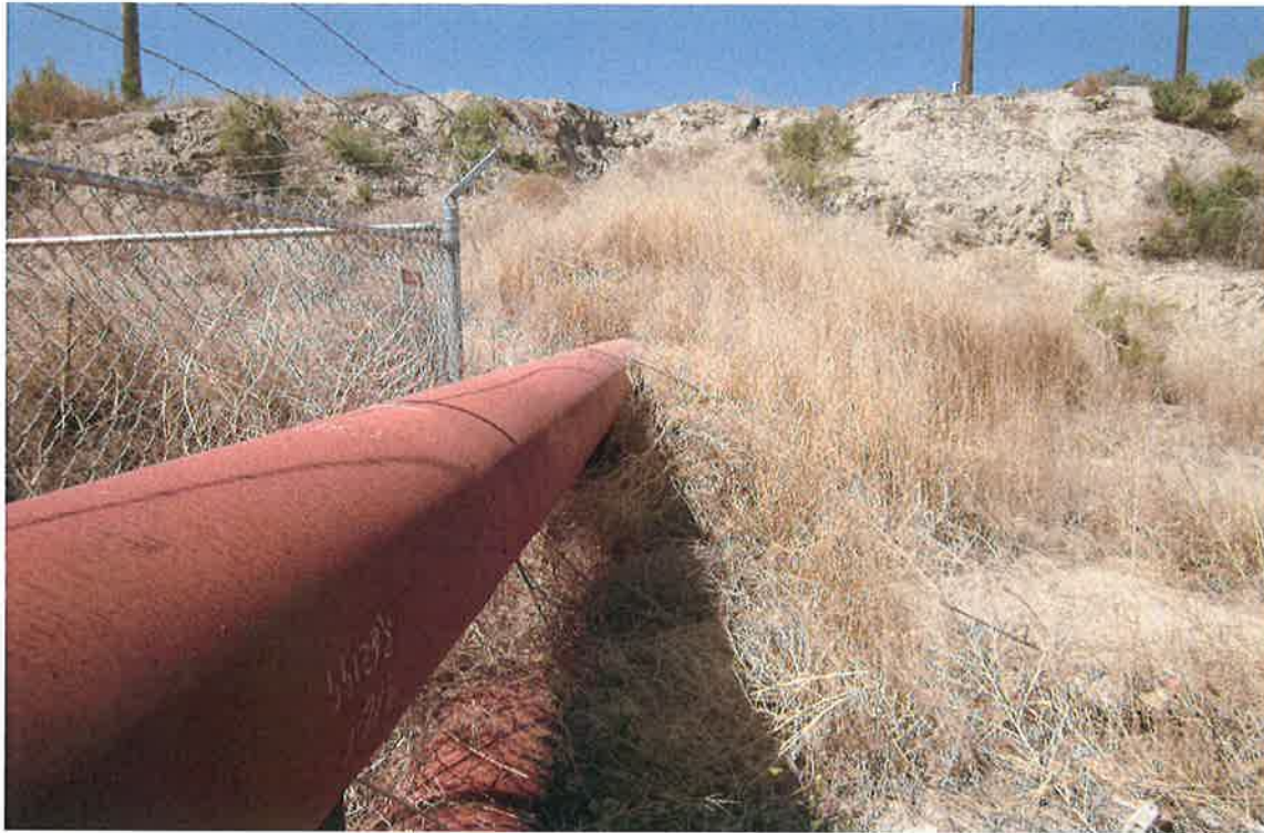
The 18" diameter pipe goes underground.
