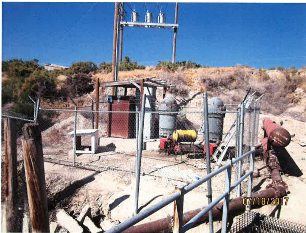
Figure 2. Photo showing the two motors. The water is diverted into the pipe closer to the ground, the larger pipe was part of the air removal system of the older diversion system.
