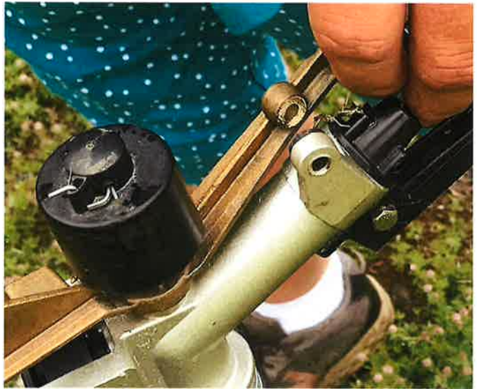
Sprinkler #2 – close up of nozzle.
