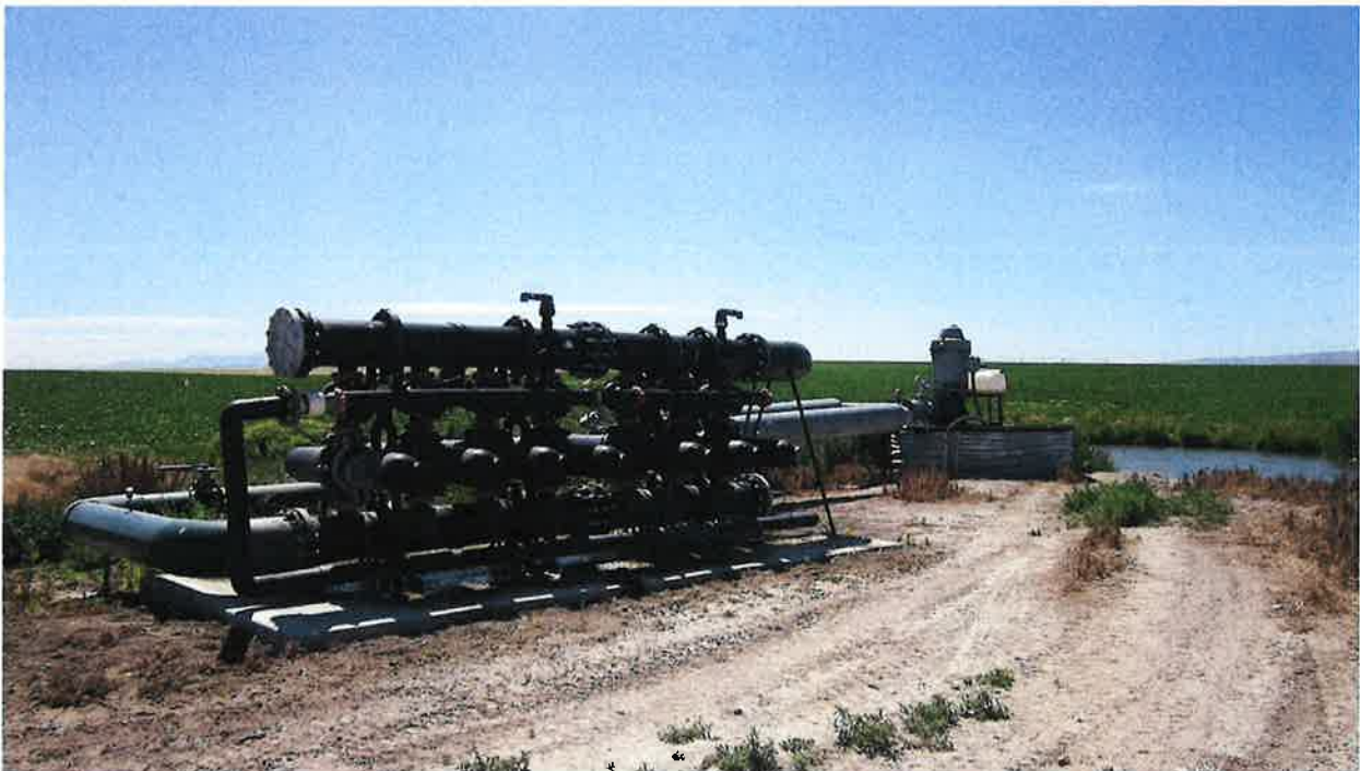
Below: Re-lift pump station to irrigation systems
