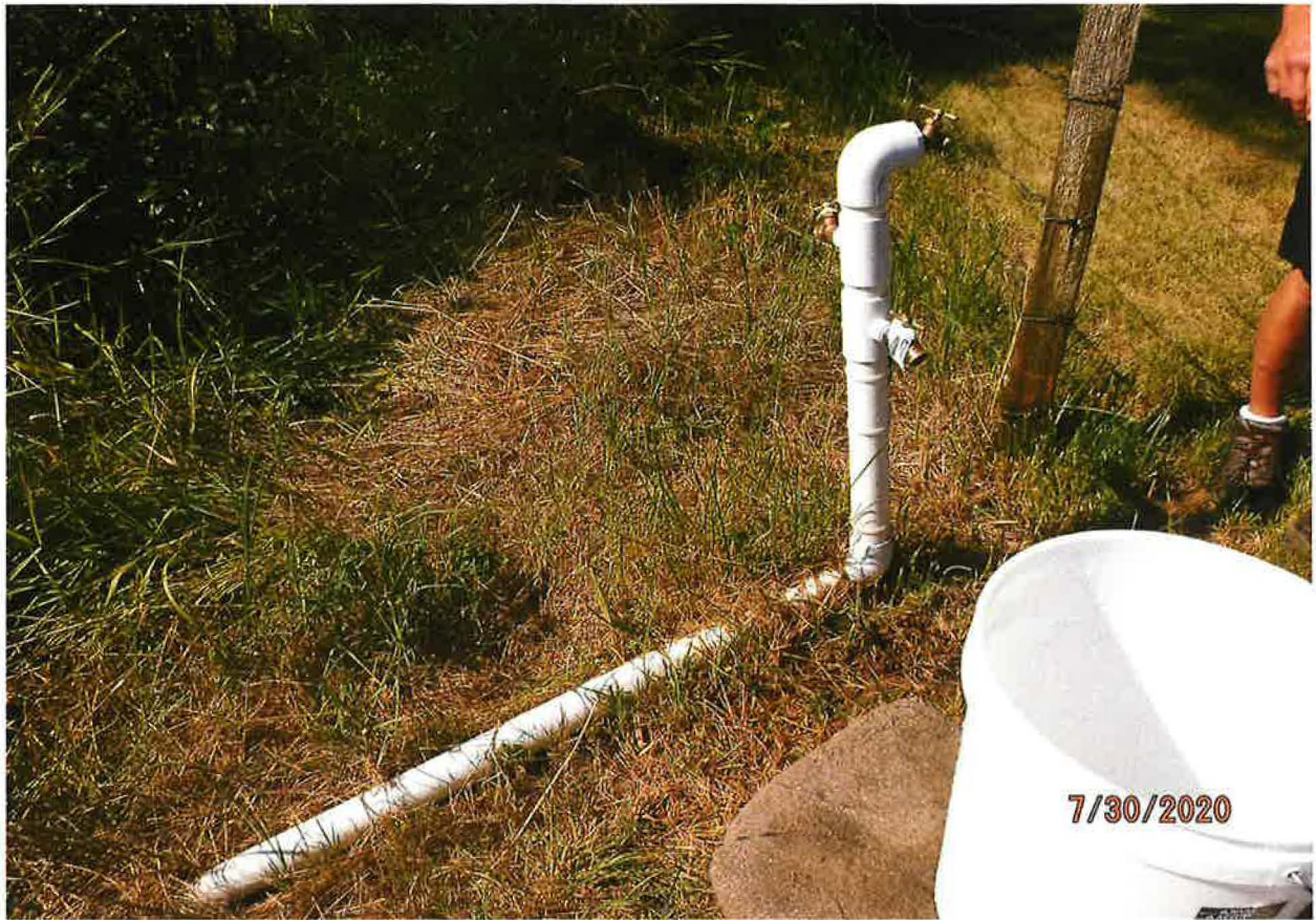
2 INCH PVC PIPE TO HOSE BIB IRRIGATION STUB WATER SYSTEM
