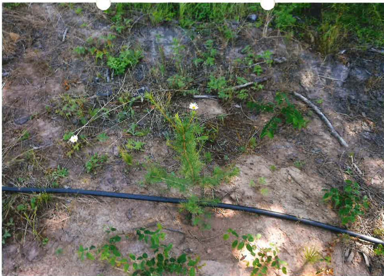
IRRIGATION 1" WATER PIPE THROUGHOUT POU
