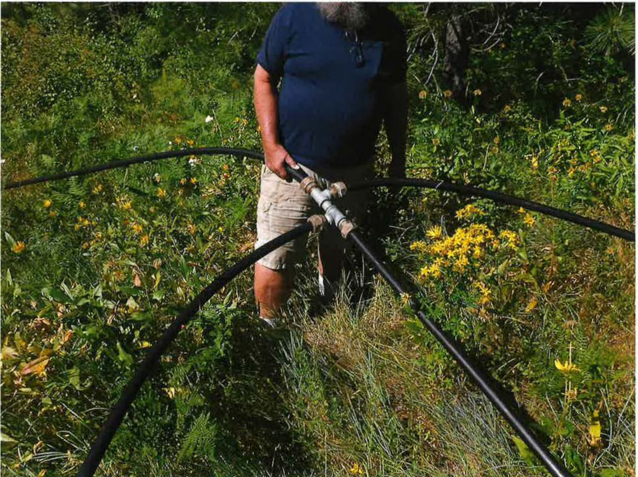
IRRIGATION SYSTEM PIPING FROM WELL TO POU
