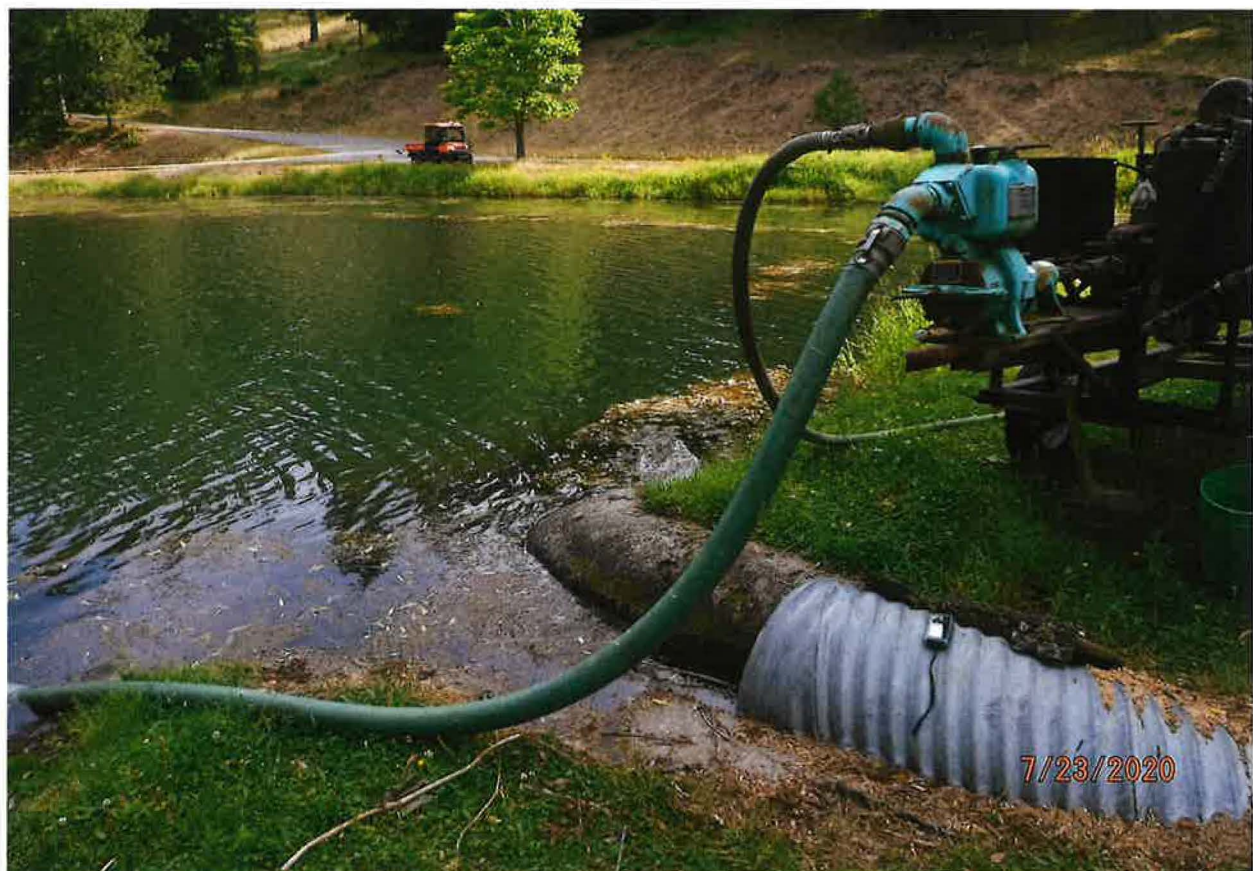
POD – GROUNDWATER & UNNAMED STREAM – OVERFLOW PIPE FROM POND TO UNNAMED STREAM CHANNEL
