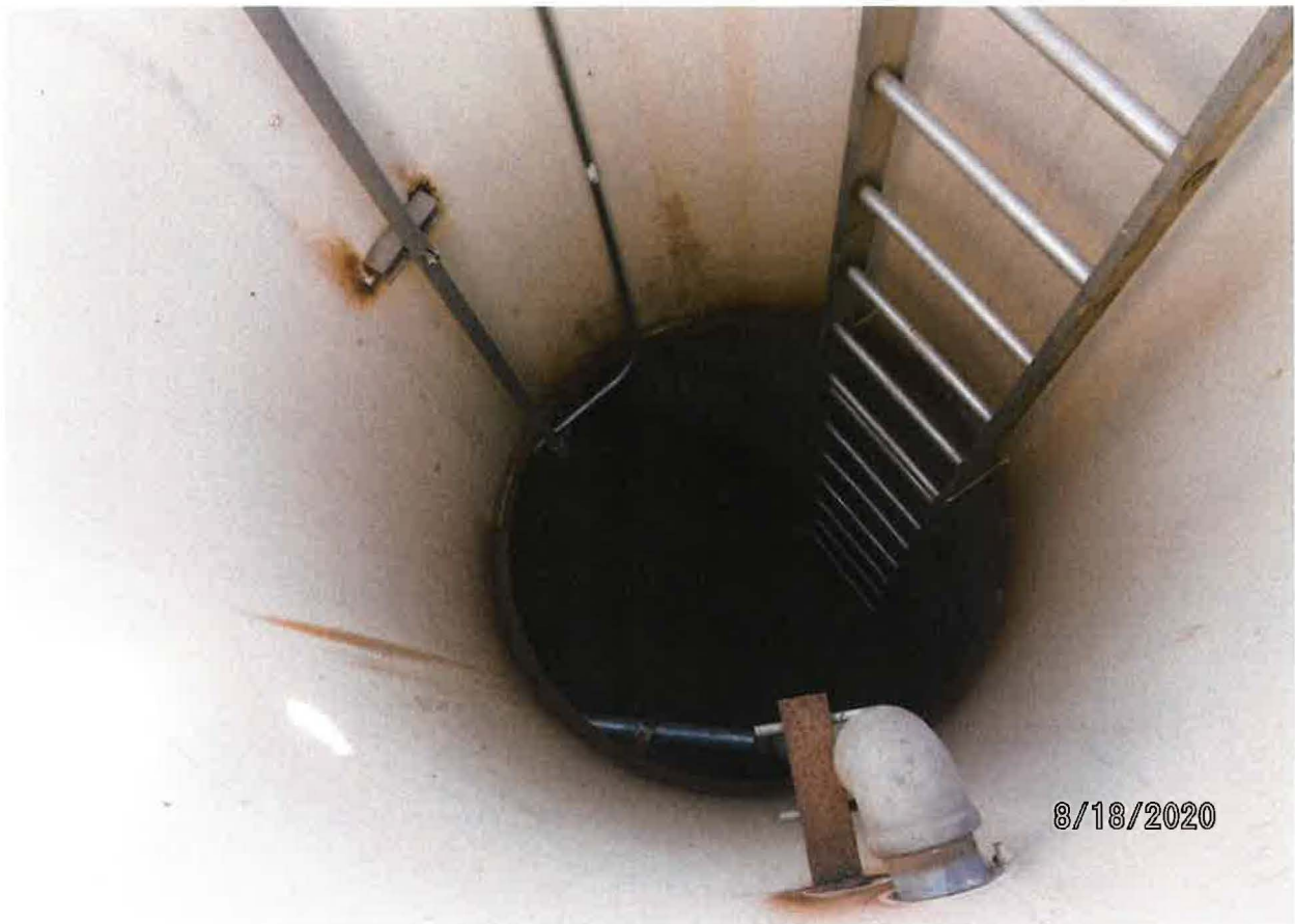
Vault containing well piping and 25 HP PUMP
