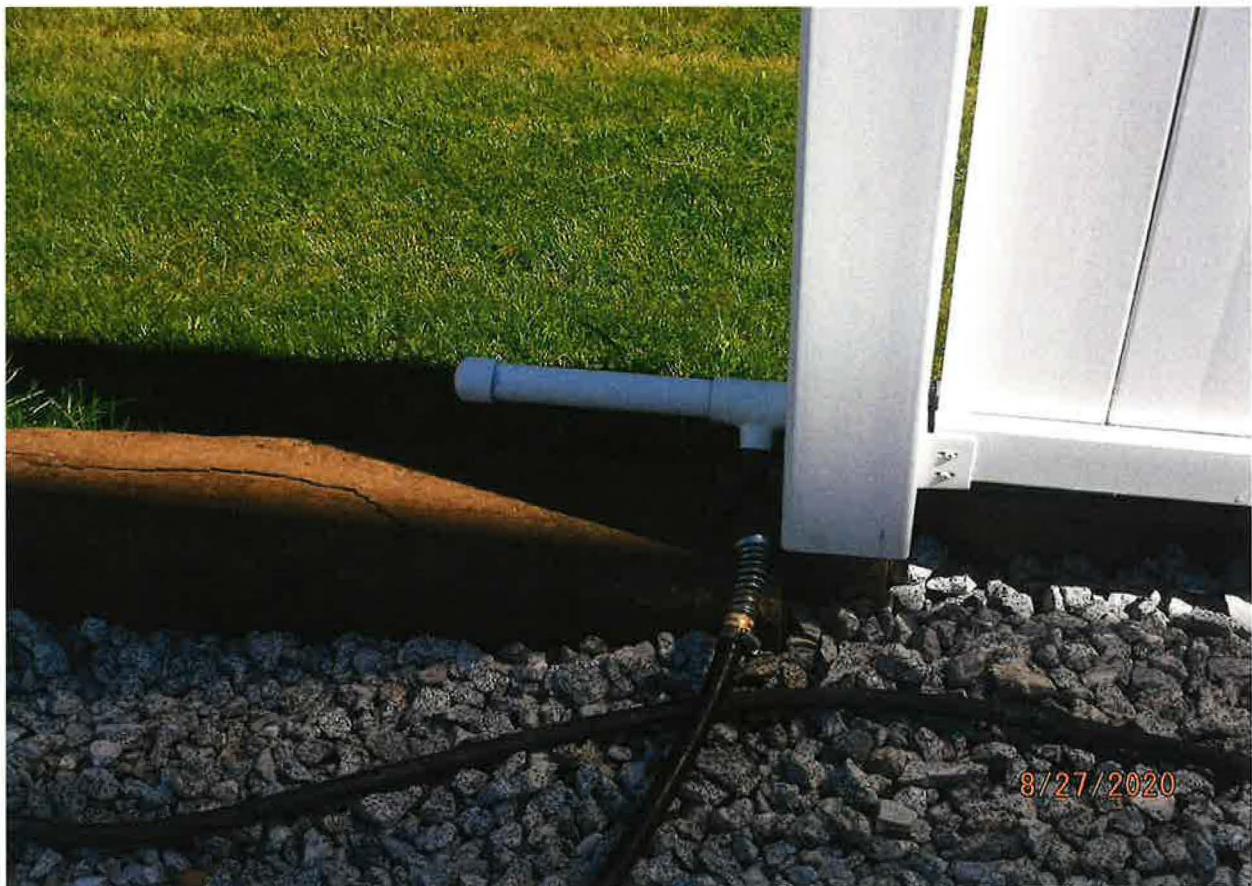
END OF IRRIGATION MAIN LINE AT POU
