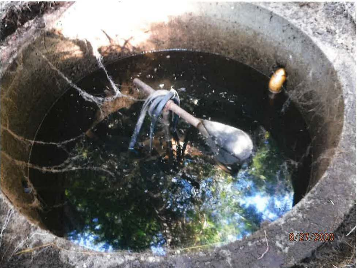
SUBMERSIBLE PUMP IN 24HR ALLOWANCE CONCRETE CISTERN
