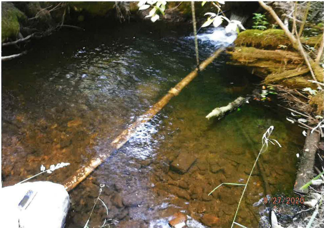
POD – PIPE WITH MESH SCREEN IN FLUME CREEK
