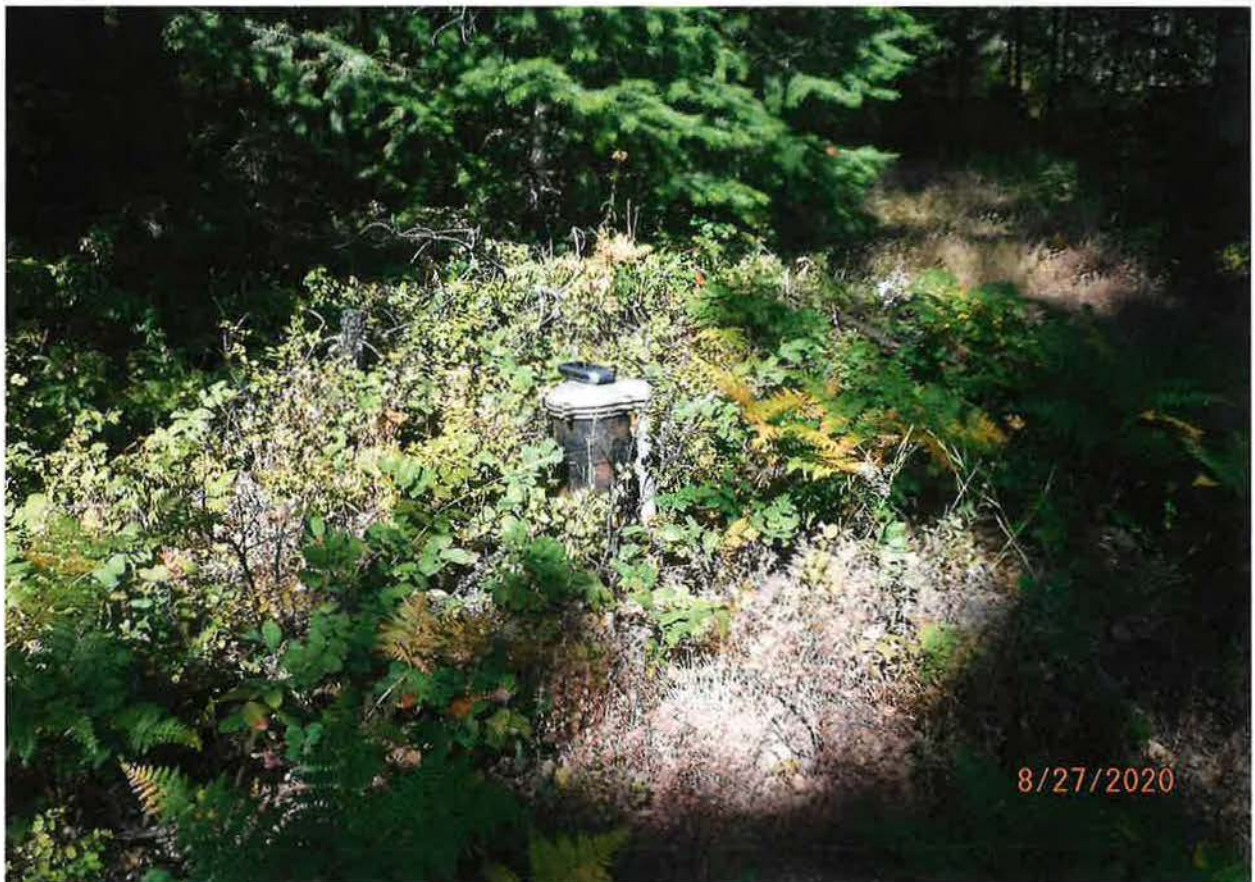
POD - WELL (96-93-N-246-000)
