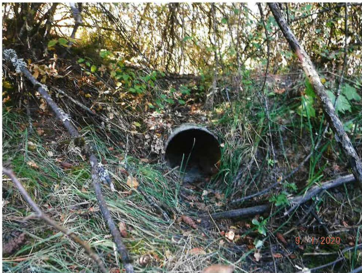
POD – EARTHEN DAM ON POND WITH OVERFLOW DISCHARGE PIPE
